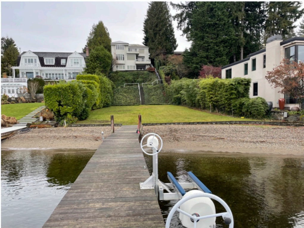
Photo 2 - Existing dock looking landward.
