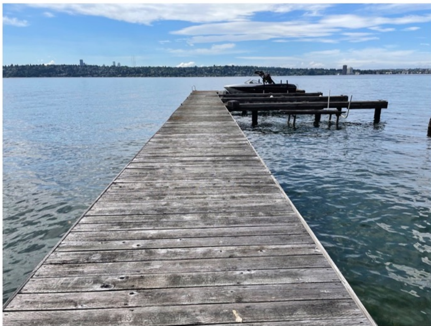
Photo 2 - Dock looking waterward.
