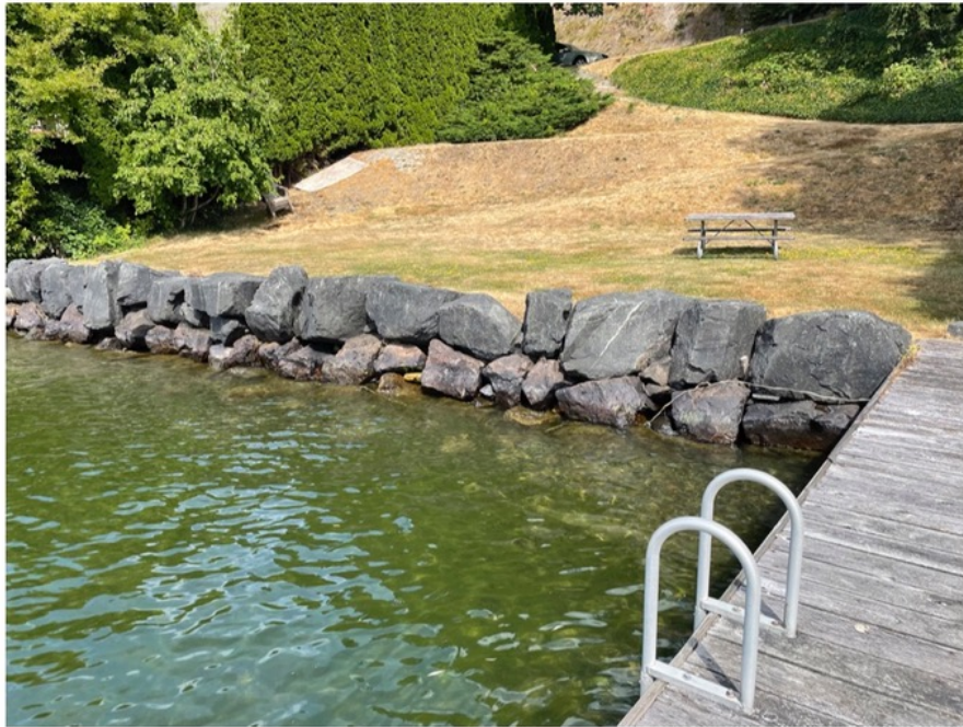
Photo 5 - Shoreline conditions at site north of dock.
