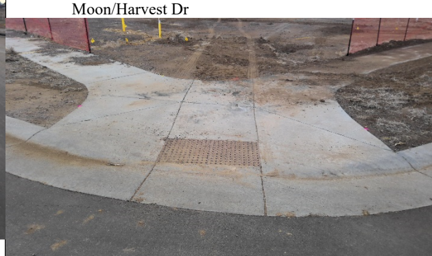
16- 2 cracks in ramp need to be sealed at Harvest Moon/Harvest Dr
