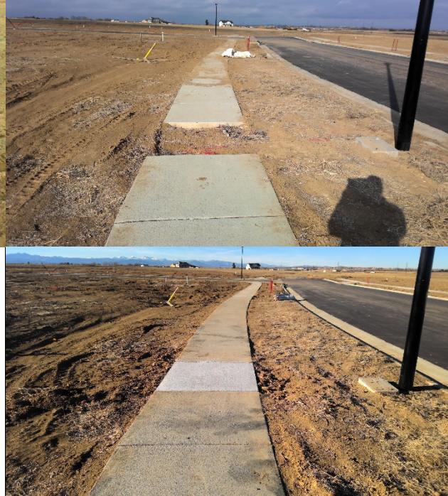
16- 2 cracks in ramp need to be sealed at Harvest Moon/Harvest Dr
