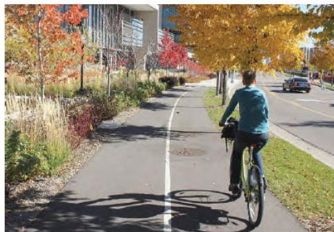
A shared use path is typically wider than a traditional sidewalk and is designed to accommodate pedestrians and cyclists.
