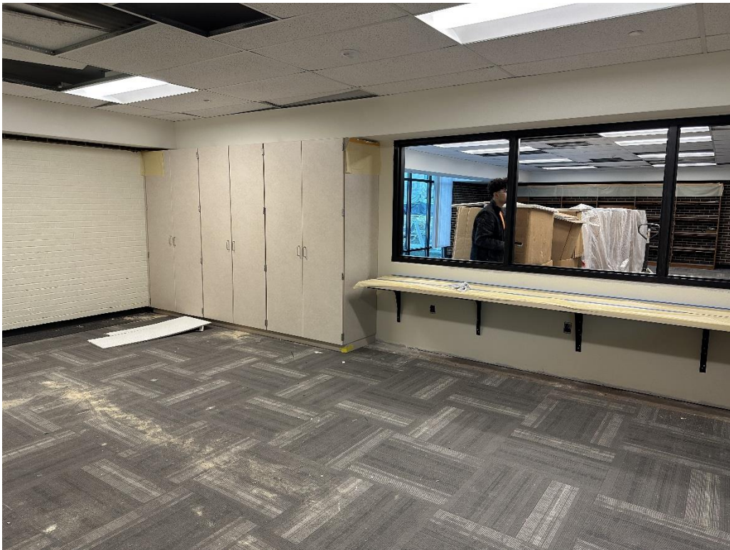
Cabinet on Left for Storage
