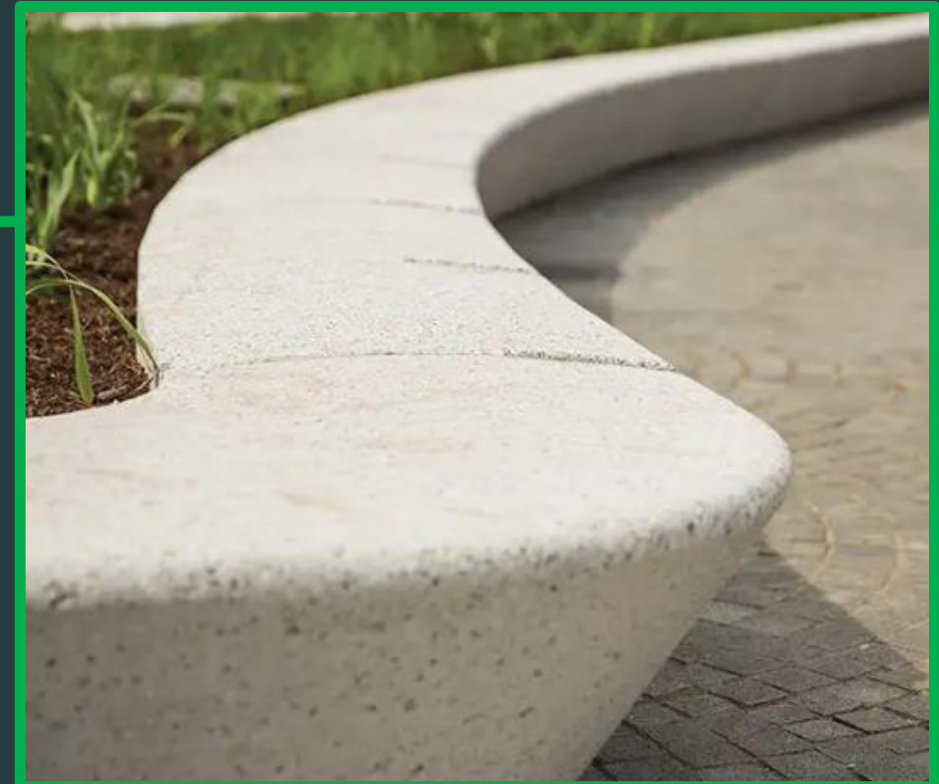
Concrete exposed aggregate seatwall
