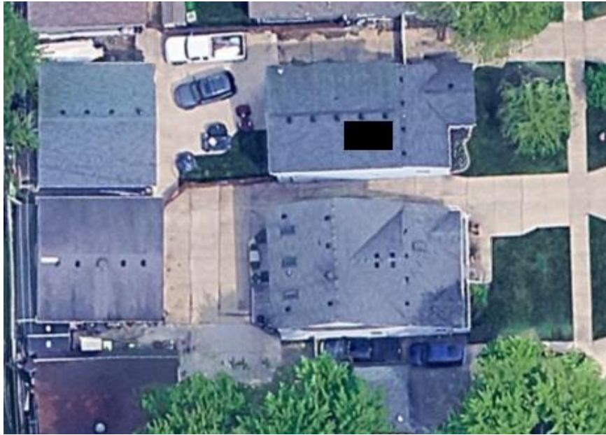
A lack of setbacks can cause sheets of water to flow onto neighboring properties.
