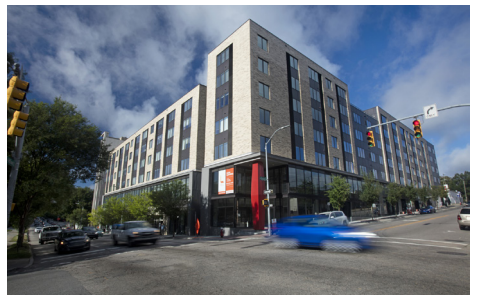
Davie Street Parking Deck | Raleigh, NC
