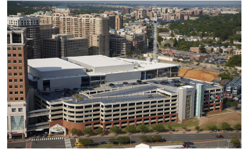
Ballston Public Parking Garage Improvements | Arlington County, VA
