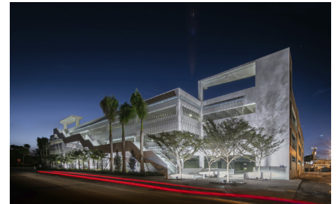
Saint Armands Parking Garage | Sarasota, FL
