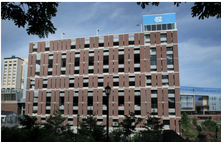
UNC-Chapel Hill Bell Tower Parking Deck and Pedestrian Bridge | Chapel Hill, NC
