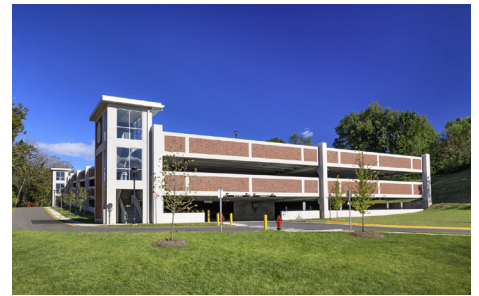
Shenandoah University Parking Garage I Winchester, VA
