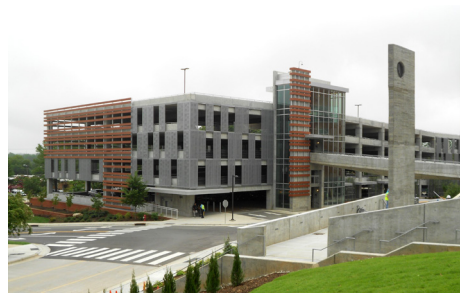
Wake Tech Health Sciences Building Parking Deck | Raleigh, NC
