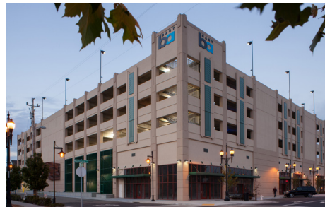
Richmond Transit Village Parking Garage | Richmond, VA
