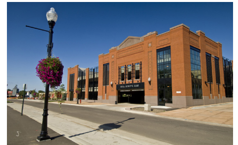
North Central Business District | Anoka, MN
