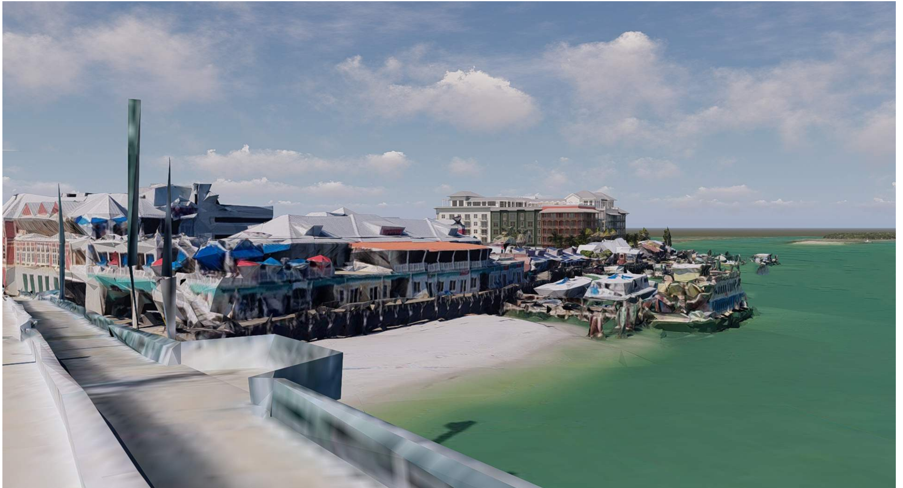
View from bridge
