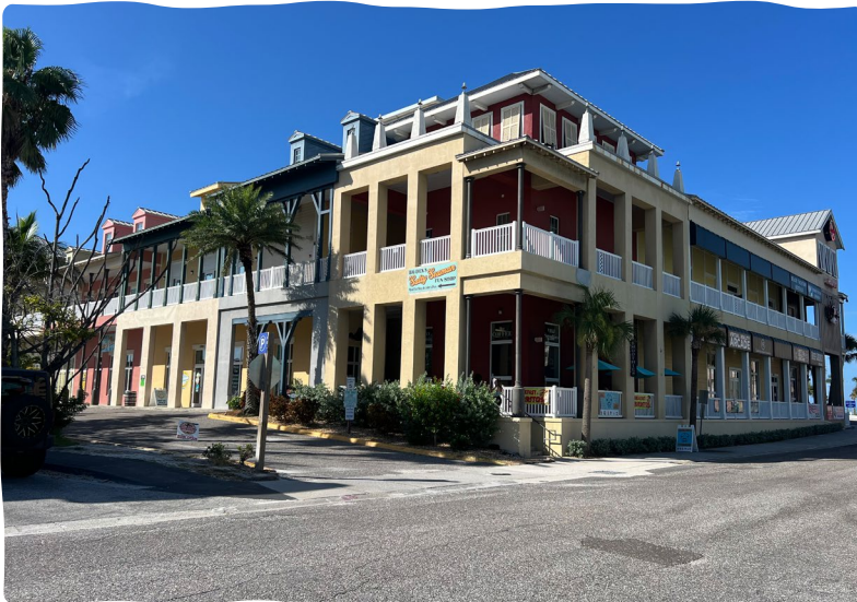
Explore additional opportunities for a public parking garage with new development that integrates retail to camouflage the parking structure.
