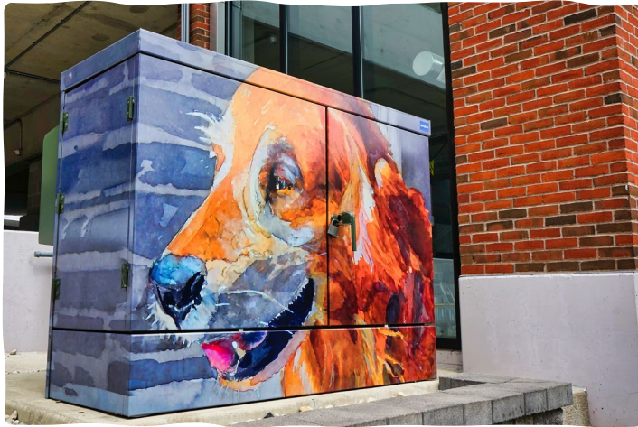
A mural program for utility boxes infuses art into the public realm
