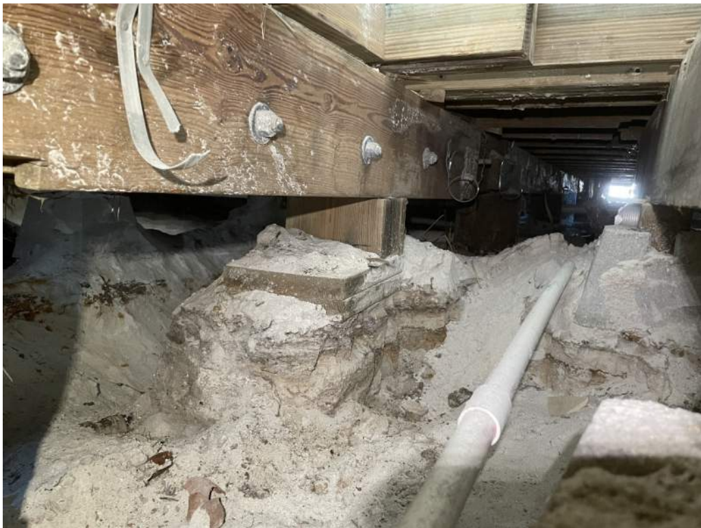
Photo 12 – Previous Retrofit of Sistered Beam
