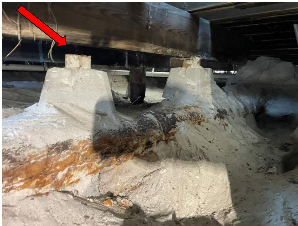
Photo 10 – Previous Retrofit with Detached Post
