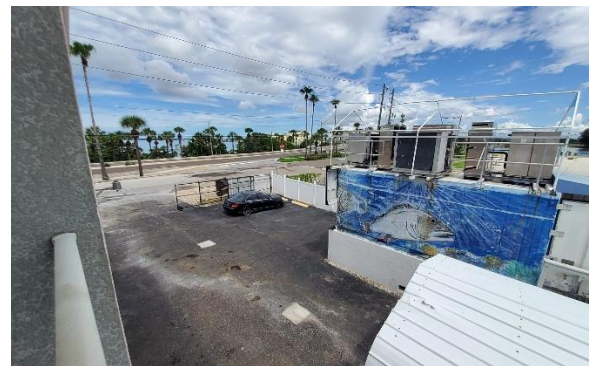
VIEW FROM BALCONY FACING NORTHWEST
