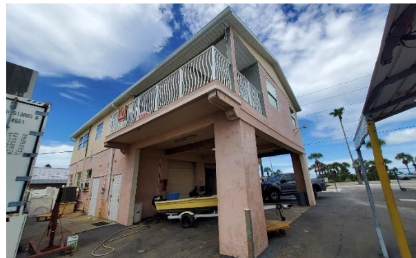
SUBJECT REAR LEFT SIDE
