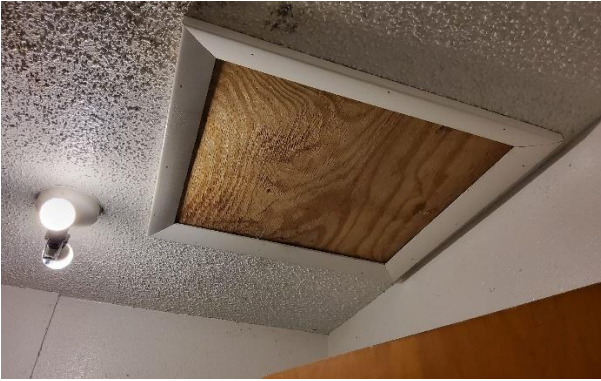
SCUTTLE TO ATTIC LAUNDRY ROOM
