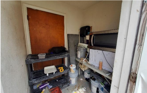
FIRST FLOOR BATH – NO FIXTURES STORAGE
