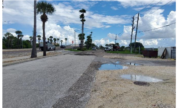
STREET SCENE ACCESS ROAD LOOKING EAST
