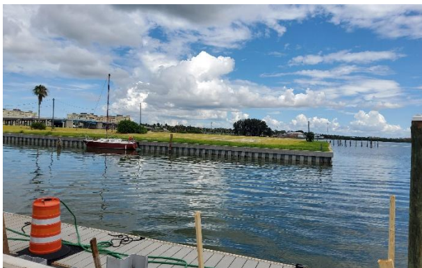
SOUTHERN EDGE OF PROPERTY LOOKING EAST
