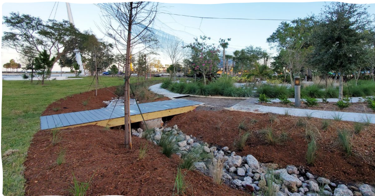
Bioswales are an attractive way to capture stormwater runoff.
