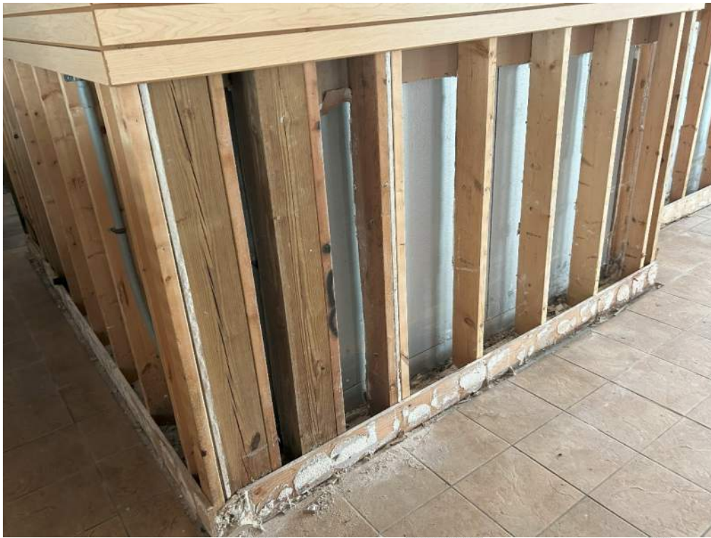
Photo 9 – View of the Interior Walls Wood Frame Structure.
