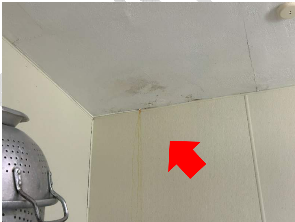
Photo 38 – Signs of Water Intrusion through in the Ceiling.
