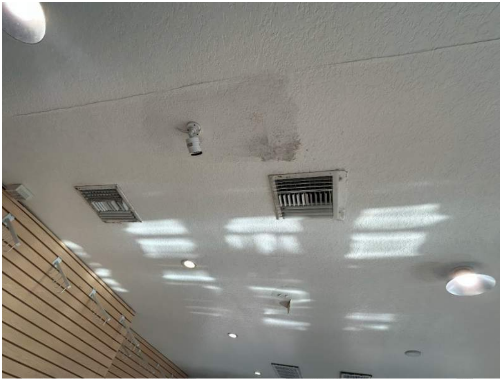
Photo 35 – Signs of Water Intrusion through the 2 nd Floor / Cracks in the Ceiling.
