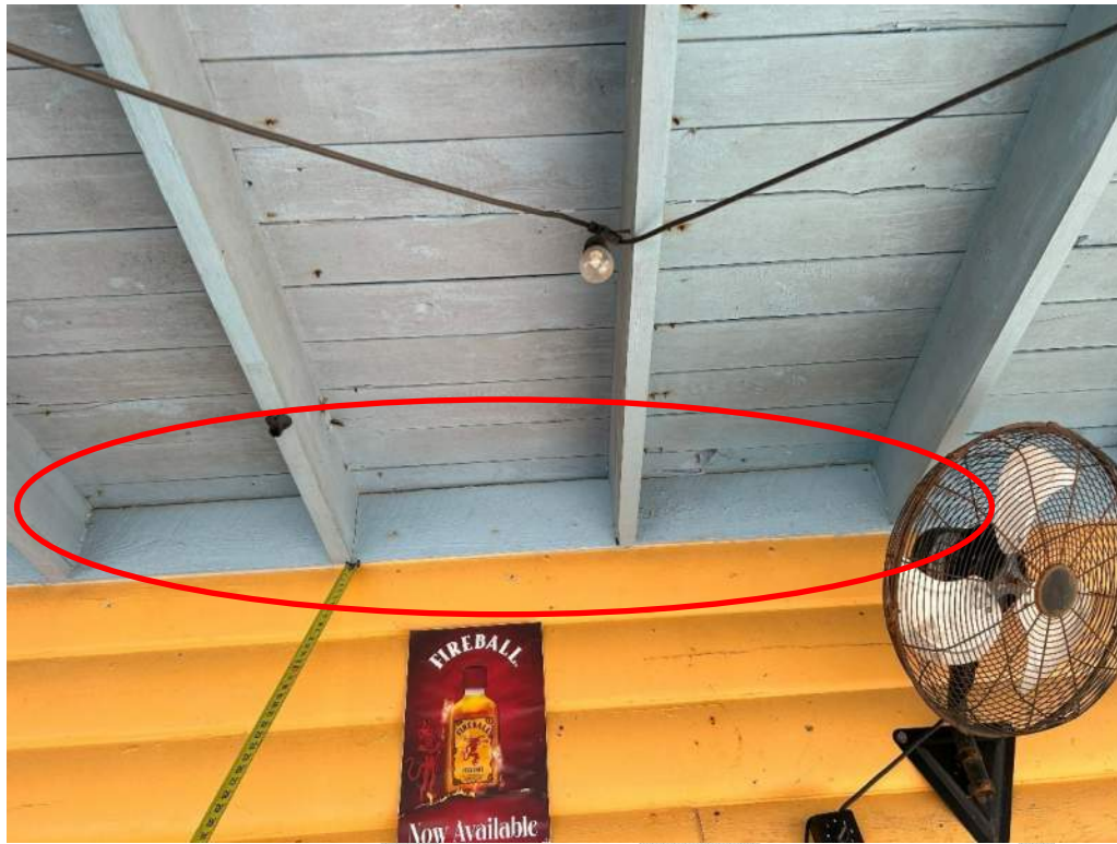
Photo 53 – Lack of Connections in the Roof Structure at Back Porch Frame.
