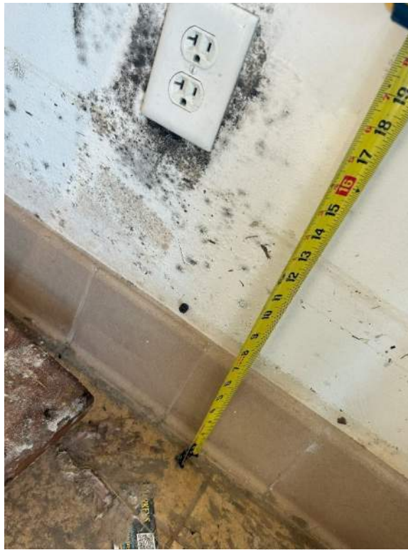
Photo 61 – Signs of Mold and Water Intrusion in the Interior of the Building (14" over finish floor).
