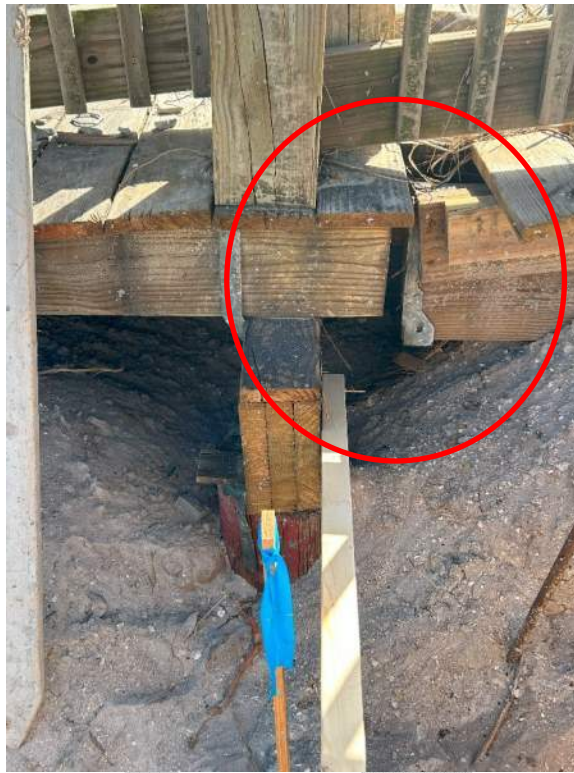
Photo 11 – Failed Connection between the Exterior Wood Deck and the Perimeter Corridor.
