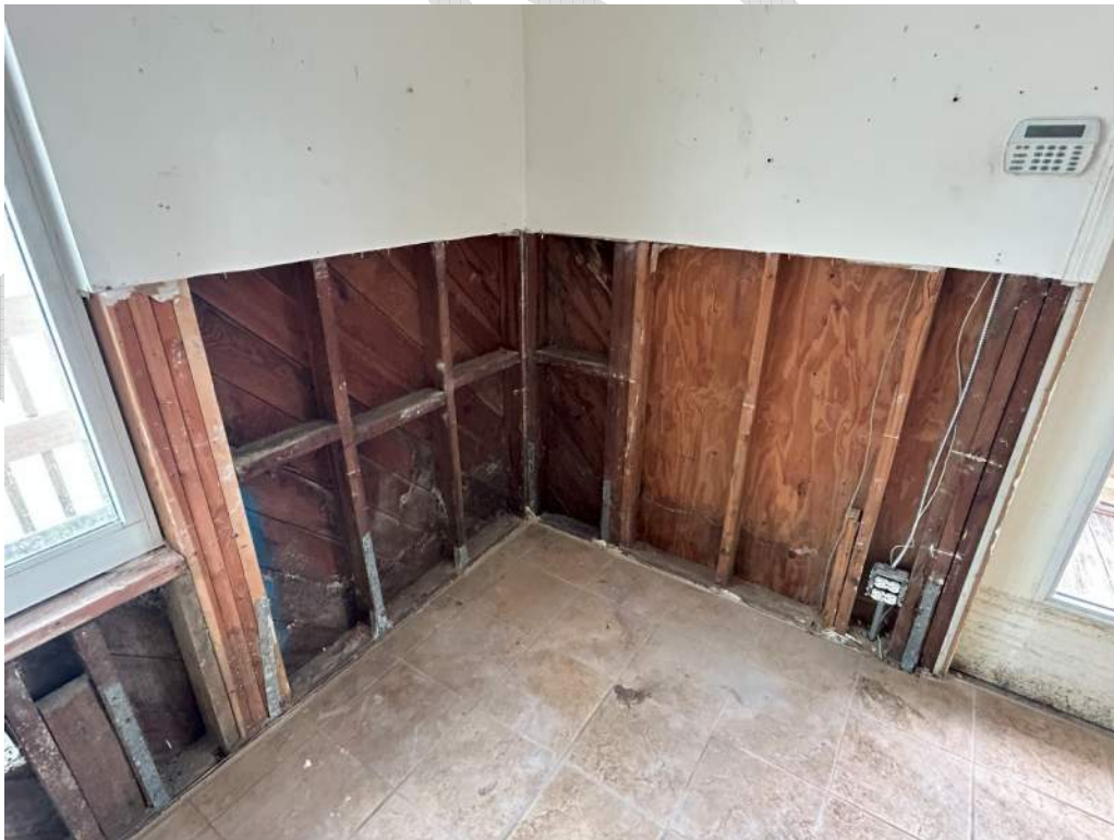
Photo 10 – View of the Exterior Walls Wood Frame Structure.
