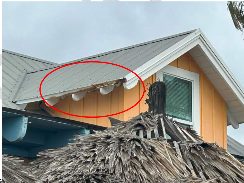
Photo 48 – Corrosion on Metal Roofing Edges.
