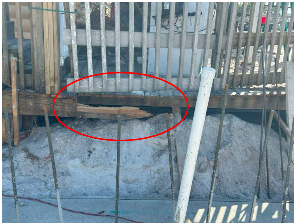
Photo 13 – Broken Exterior Wood Beam at the Outside Deck (in December 2024).
