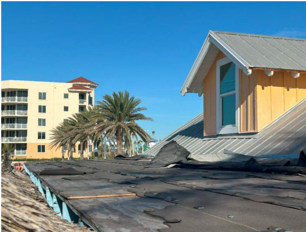
Photo 49 – Outside View of Built-up Roofing Destroyed.
