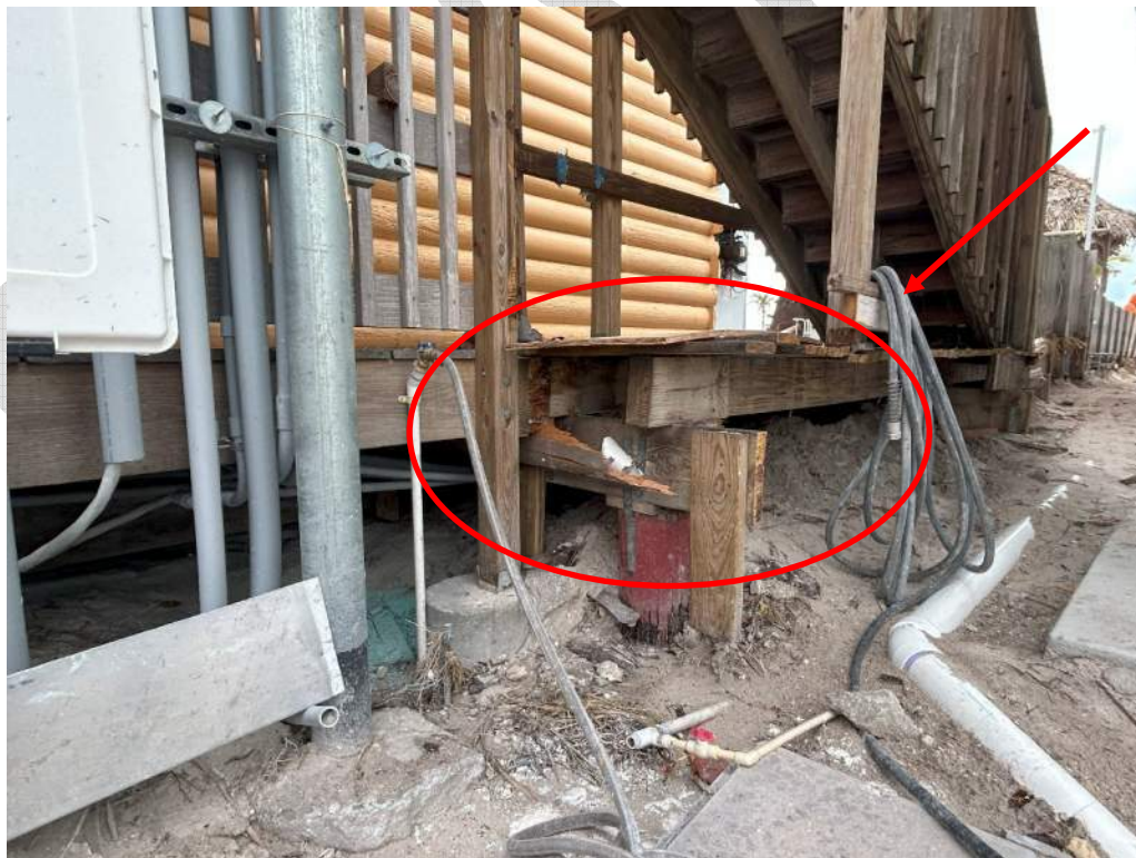
Photo 13 – Broken Exterior Wood Beam at the Outside Deck (in December 2024).
