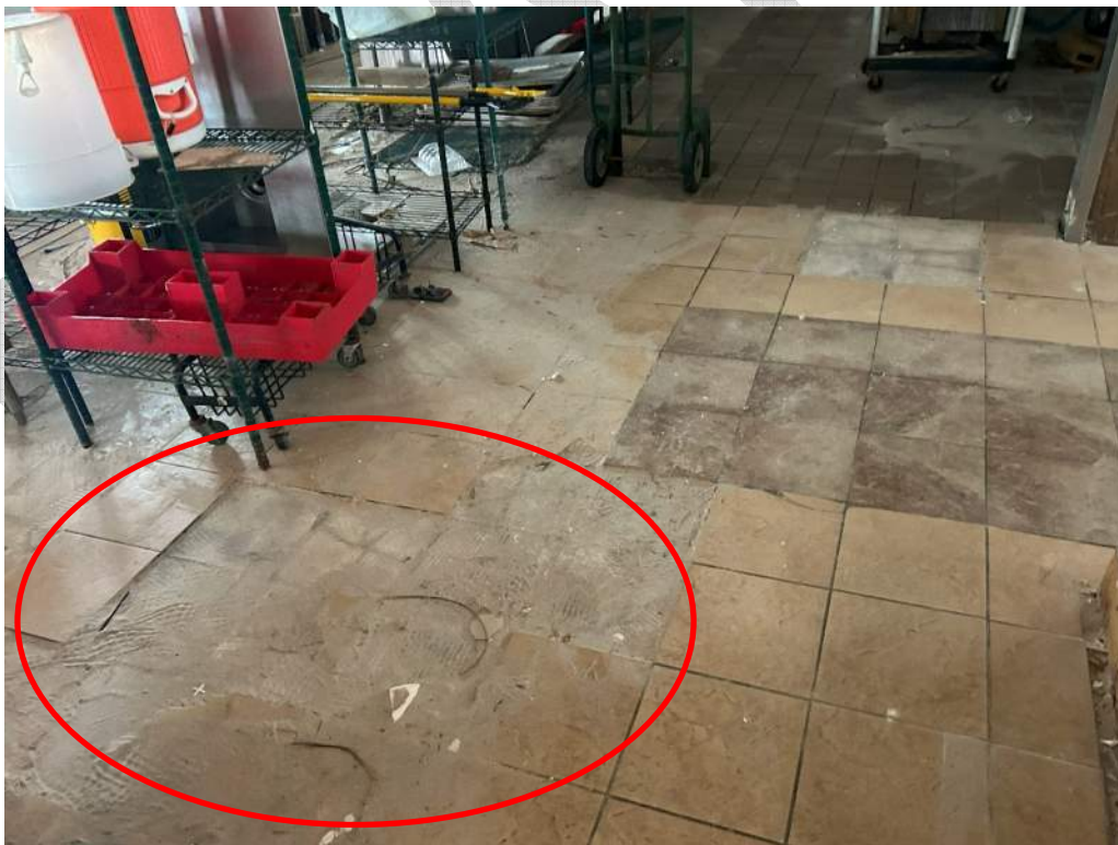
Photo 16 – One of the Areas with Possible Floor Depression
