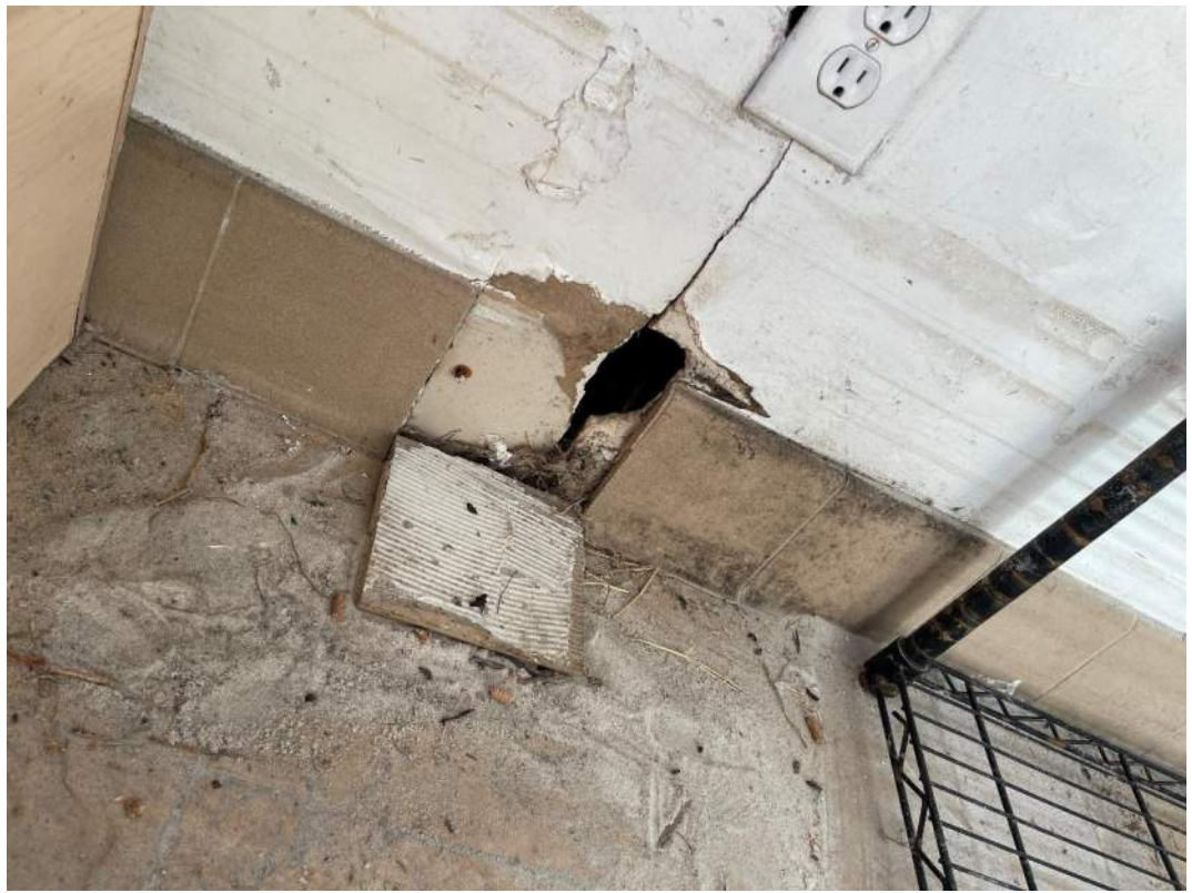
Wall base, hole in wall cavity with water intrusion.
