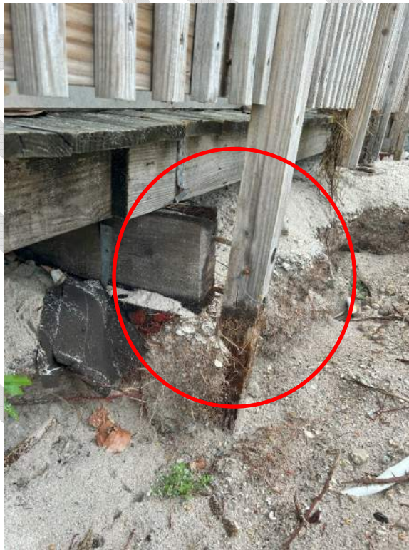
Photo 12 – Failed Connection between the Beam that support the Southeastern Perimetral Corridor and the Wood Column that Support its Wooden Handrail (its bottom is rotten).
