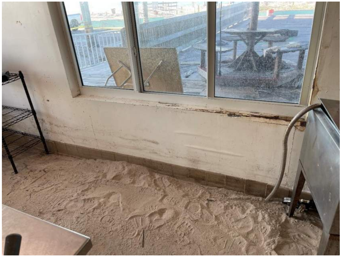
Sand/water intrusion in walls.
