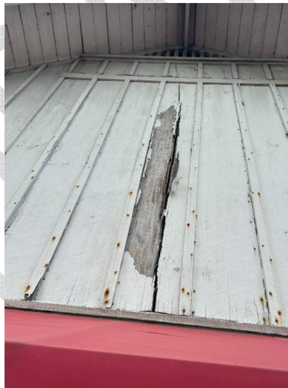
Photo 44 – Close Up View of Exterior Siding Broken at Southeast façade of 2 nd Floor (Attic), also Note Wooden Nails Corroded.
