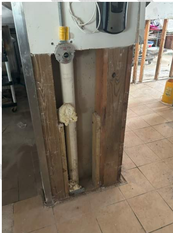
Photo 8 – View of one of the Interior Intermediate Double Columns of the Walls Wood Frame Structure.
