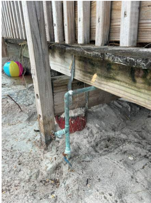
Photo 5 – View of one of the Foundation Piles that support the Perimetral Hallway.
