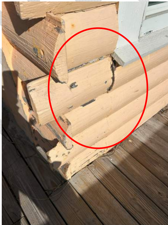
Photo 20 – Minor Signs of Possible Movement in SE Corner of the Building.
