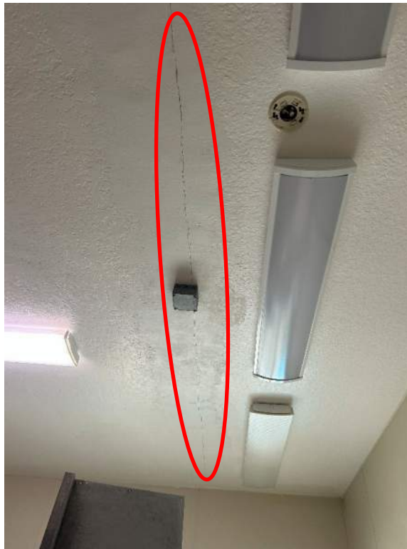
Photo 37 – Signs of Water Intrusion through the Ceiling and Longitudinal Crack in a Wood Truss direction.
