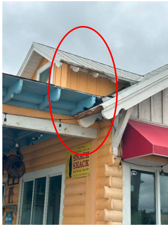
Photo 47 – Corrosion on Metal Roofing Edges.
