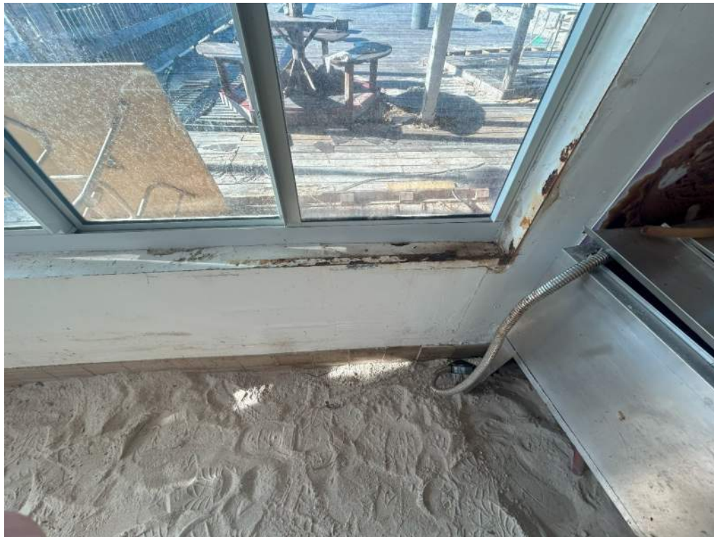
Photo 59 – Corrosion in Metal Corner Beads of Interior Walls.
