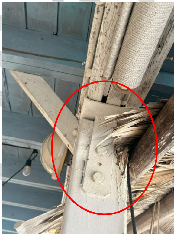
Photo 54 – Top of one of the Wood Column of the Back Porch that was Impacted by Outside Tikis.
