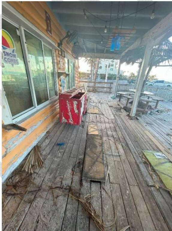
Photo 58 – Wooden Boards Loose at the Back Porch.
