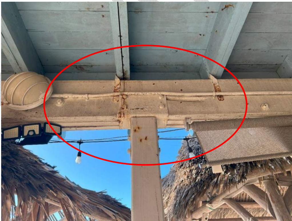
Photo 52 – Corroded Connections at Back Porch Frame.
