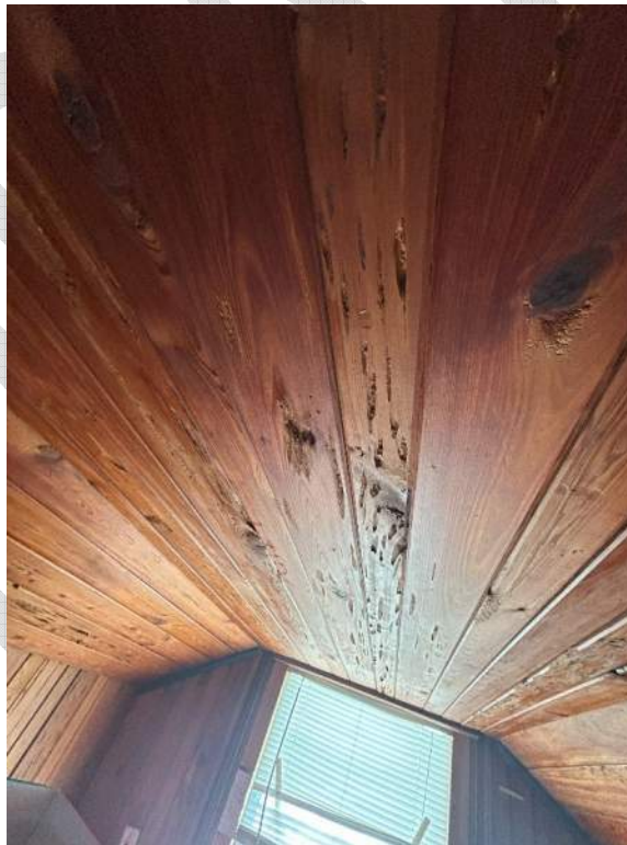
Photo 42 – Termite Damages in Wood Ceiling of the Attic.
