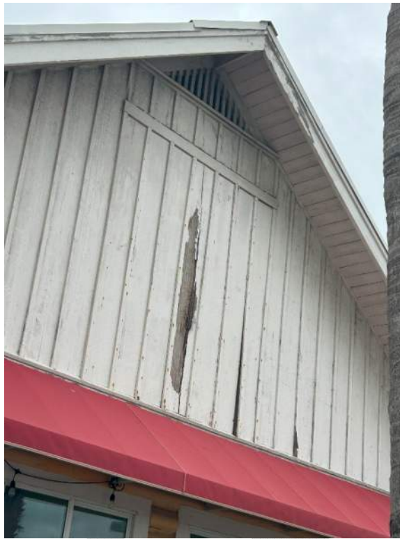
Photo 43 – Exterior Siding Broken at Southeast Façade of 2 nd Floor (Attic).
