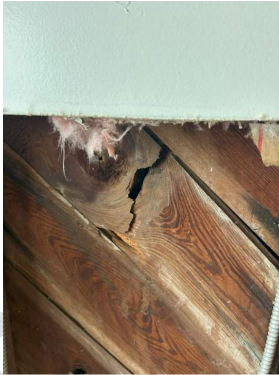
Photo 27 – Broken Wood Board of the Exterior Wall Sheathing of the Cabin Wood Frame.
