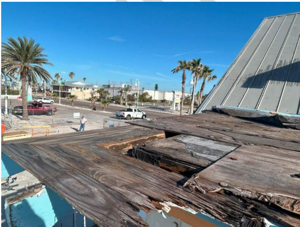
Photo 50 – Back Porch Roof Frame and Sheathing Destroyed.
