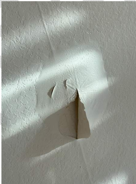
Photo 36 – Signs of Water Intrusion through in the Ceiling
