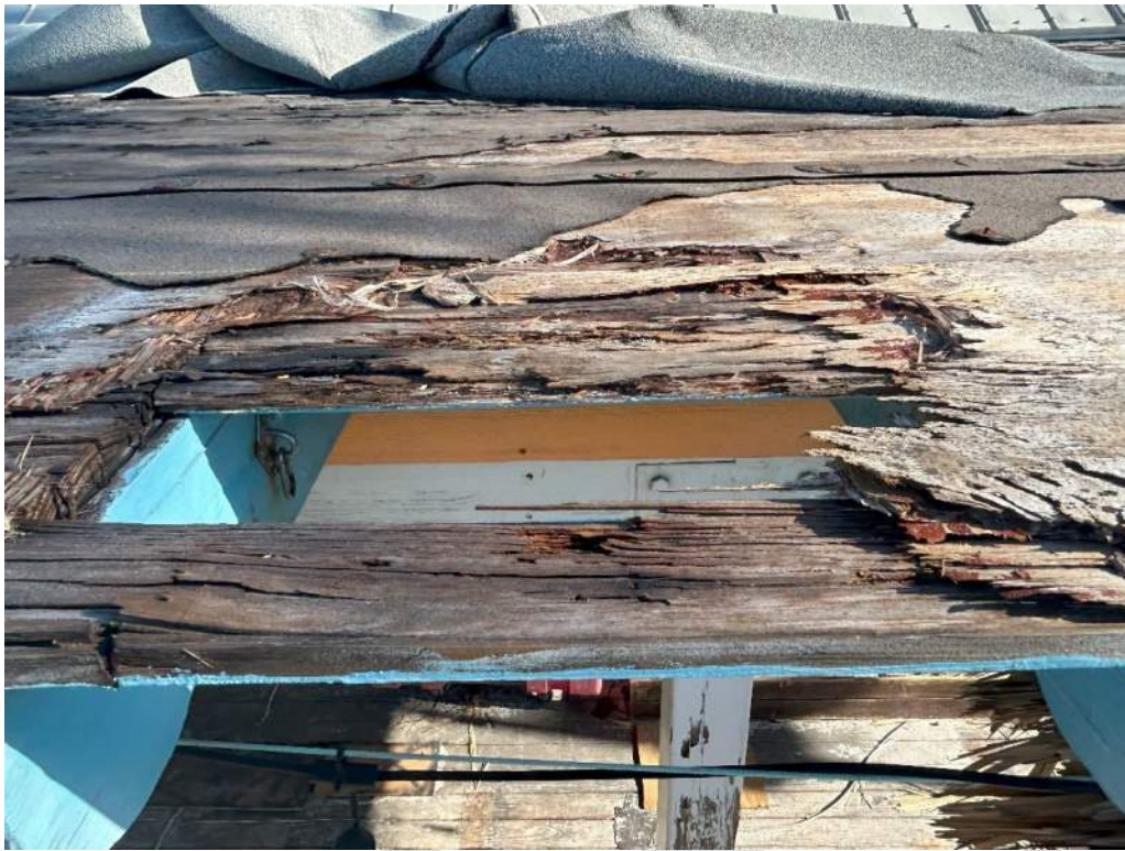
Photo 51 – Back Porch Roof Sheathing Destroyed.
