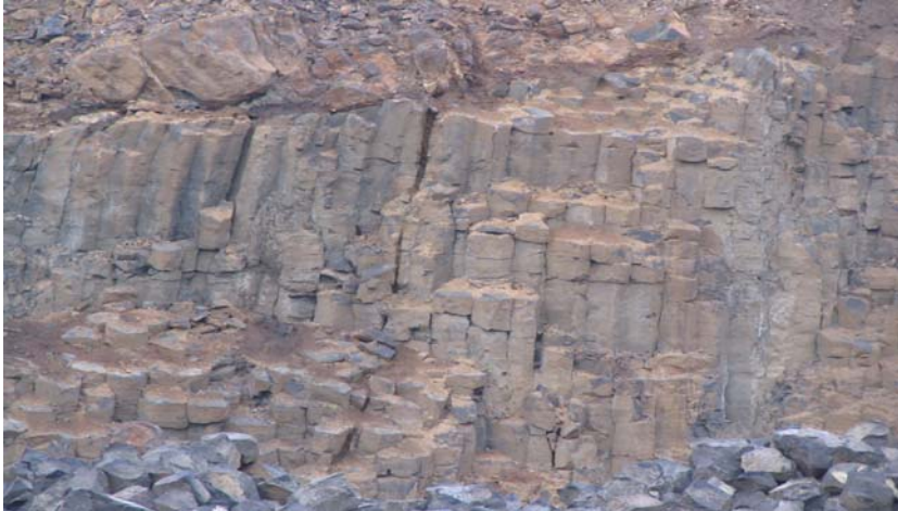
Basalt quarries in the upper watershed showing fractures
