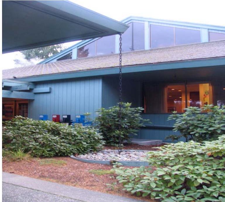
Infiltration and recharge of roof runoff into stone infiltration chambers via “rain chains”
