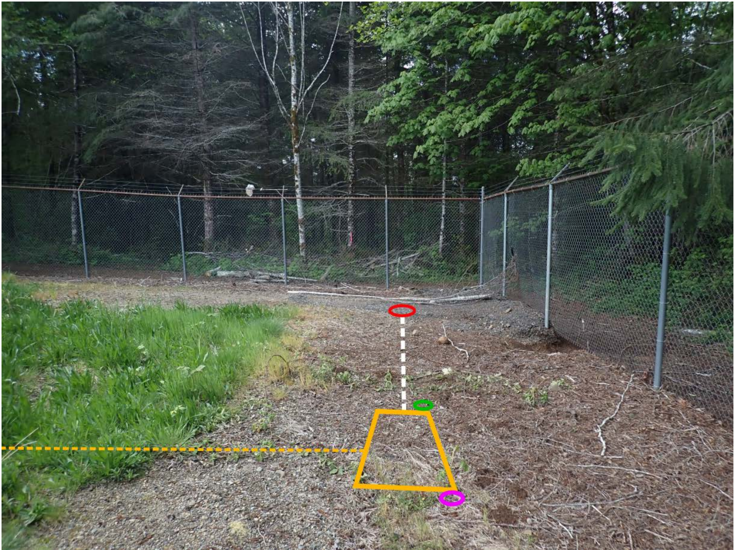
Image 6: Looking west at the station configuration for 1207-DOORS. The post-hole sensor (marked by red circle) will be located in the northwest corner of the fenced-in utility compound. The post and power enclosure (marked by the orange rectangle) will be located approximately 20 ft to the east of the post-hole sensor, along the north fence line of the utility compound. Cabling (dashed white lines) between the sensor and the post and power enclosure will be trenched. Power for the instrument will be provided by an outdoor pole-mounted 120v AC connection located approximately 16m to the southeast. AC power will be converted to low-voltage DC current and trenched to the post and power enclosure (orange dashed line). The trench path for the low-voltage power cable will depend on the location of buried utilities (fiber). A GPS antenna (green circle) will be mounted to the post and power enclosure. A Nanobeam puck (purple circle) will be mounted to the post and power enclosure and pointed to the comms shack in the northeast corner of the fenced-in utility compound where contractors will mount a second Nanobeam puck.
