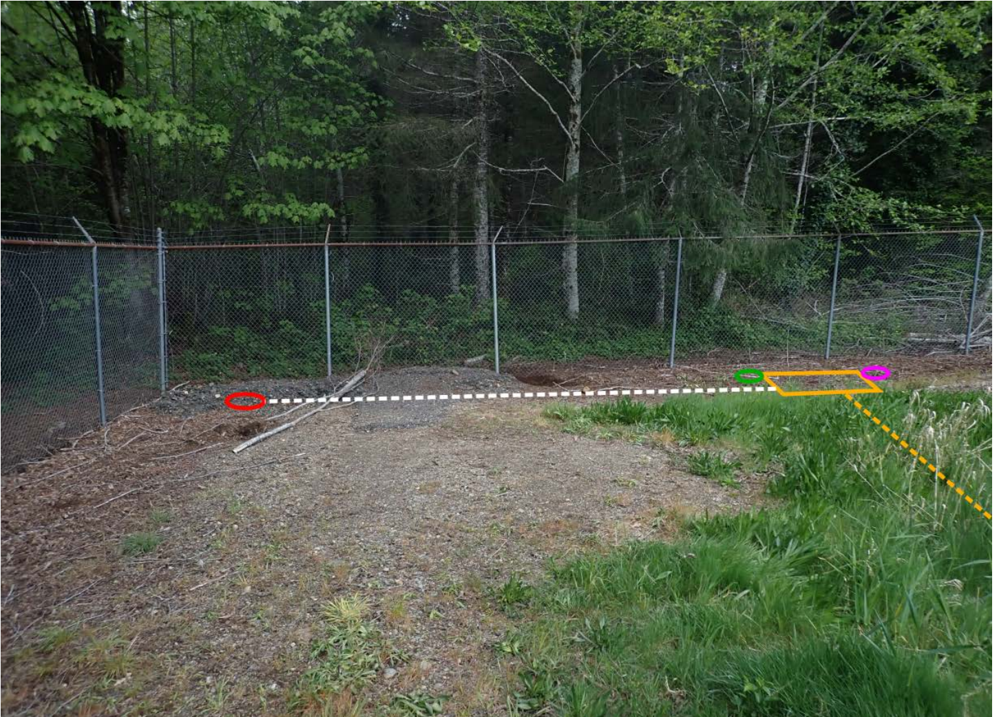
Image 5: Looking north at the station configuration for 1207-DOORS. The post-hole sensor (marked by red circle) will be located in the northwest corner of the fenced-in utility compound. The post and power enclosure (marked by the orange rectangle) will be located approximately 20 ft to the east of the post-hole sensor, along the north fence line of the utility compound. Cabling (dashed white lines) between the sensor and the post and power enclosure will be trenched. Power for the instrument will be provided by an outdoor pole-mounted 120v AC connection located approximately 16m to the southeast. AC power will be converted to low-voltage DC current and trenched to the post and power enclosure (orange dashed line). The trench path for the low-voltage power cable will depend on the location of buried utilities (fiber). A GPS antenna (green circle) will be mounted to the post and power enclosure. A Nanobeam puck (purple circle) will be mounted to the post and power enclosure and pointed to the comms shack in the northeast corner of the fenced-in utility compound where contractors will mount a second Nanobeam puck.
