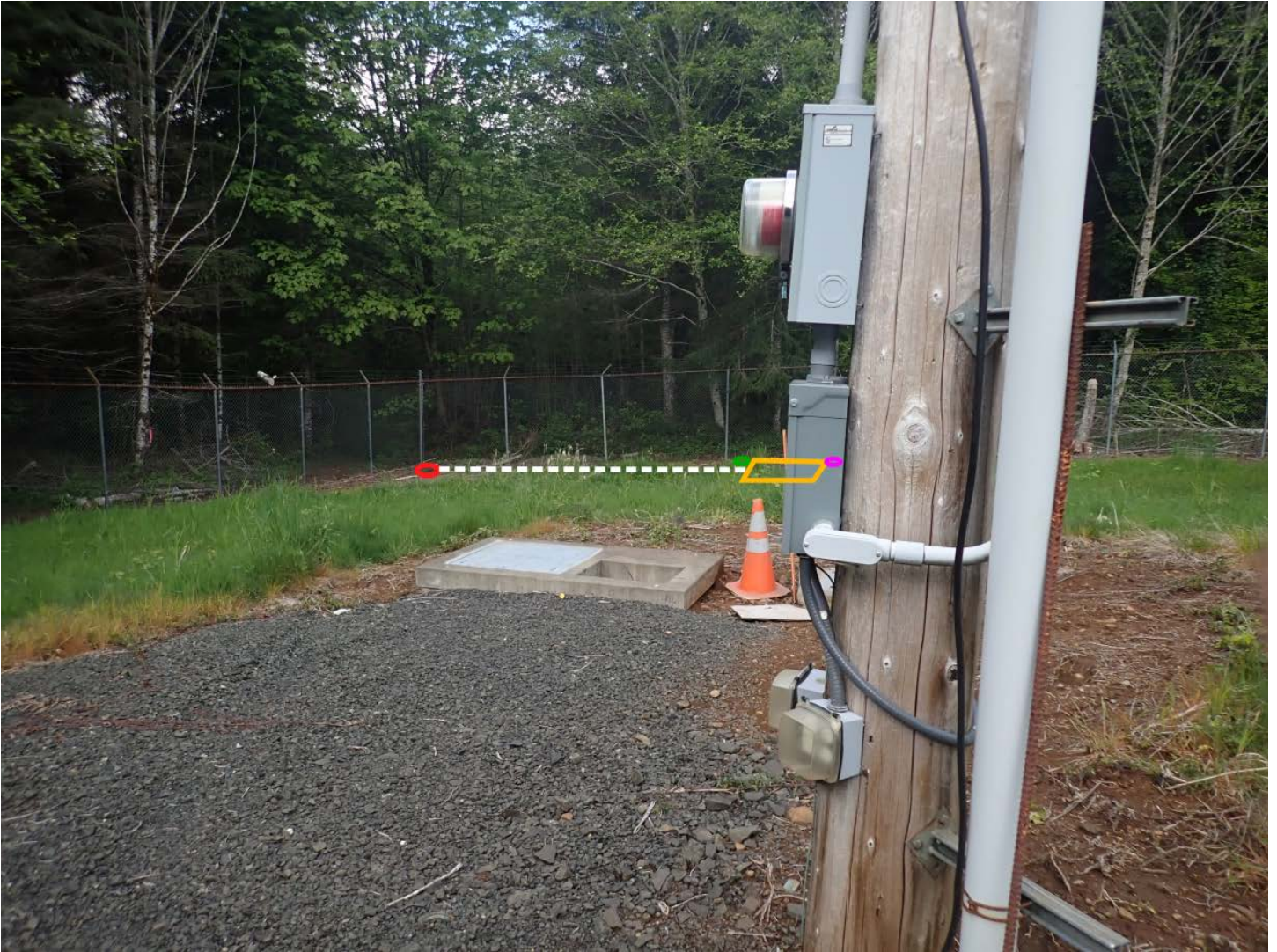
Image 8: Looking north northwest at the AC power pole that will provide power for the instrument. The proposed station location is depicted in the background of the image. AC power will be converted to low voltage DC power and trenched to the post and power enclosure. The precise path of trenching will depend on the location of other buried utilities (fiber). A small repeater box will need to be mounted to the power pole to host the AC to DC power converter. An electrician will need to be onsite to pull power from the power pole.
