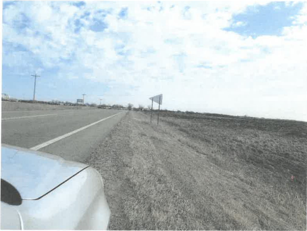
View West along T.H. 68
