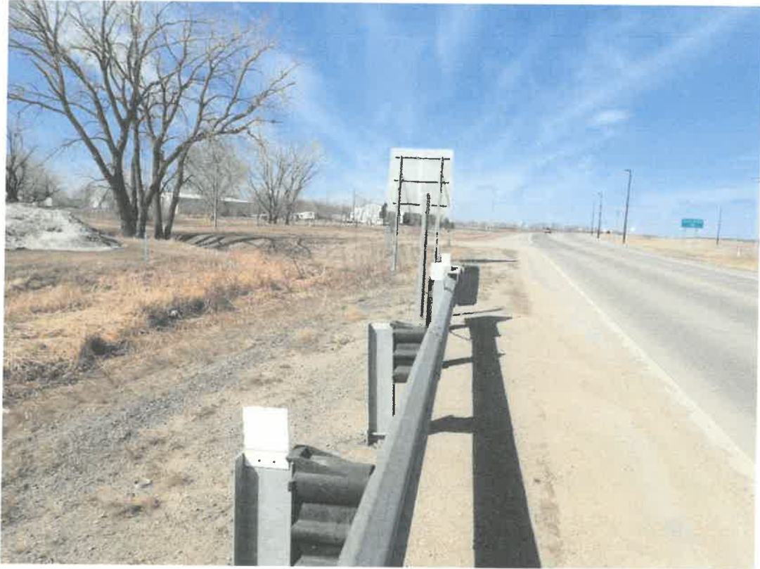
View West along T.H. 68
