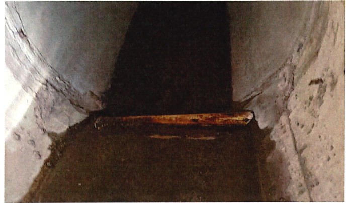
H - Hole @ 2.4 ft. large hole in pipe, can see storm sewer line in hole
