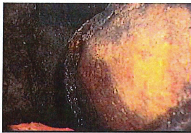
H - Hole @ 2.4 ft. large hole in pipe, can see storm sewer line in hole
