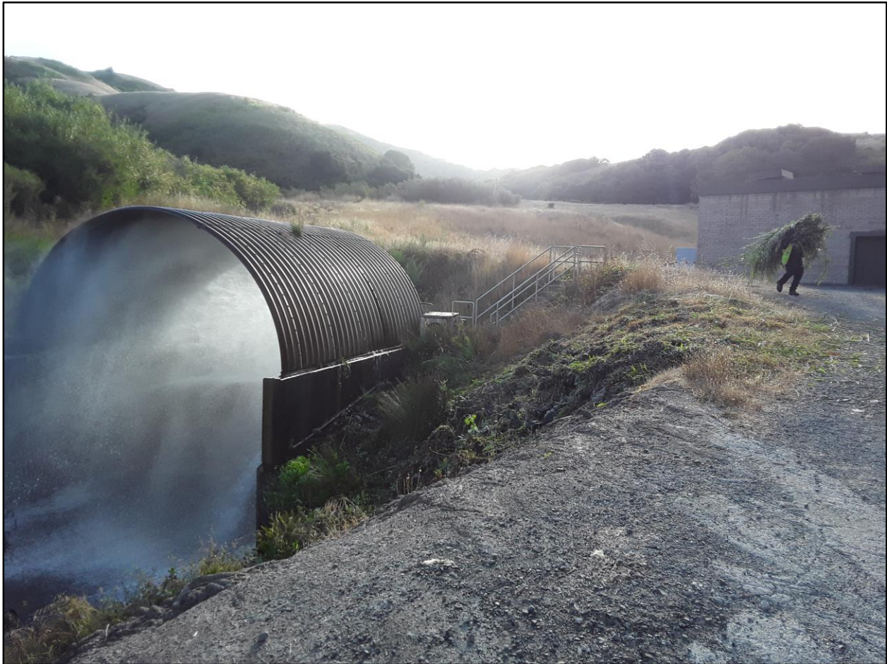
Photo 20: Facility Maintenance at the Soulajule Dam
