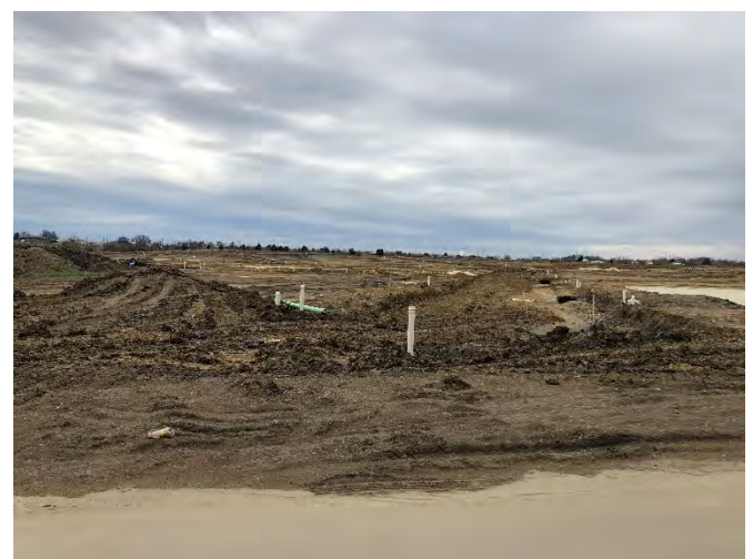
Land under construction in Phase II
