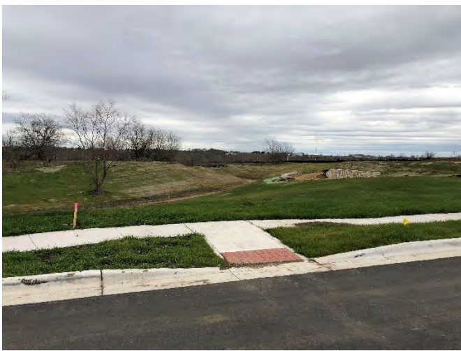
View of completed improvements in Phase I
