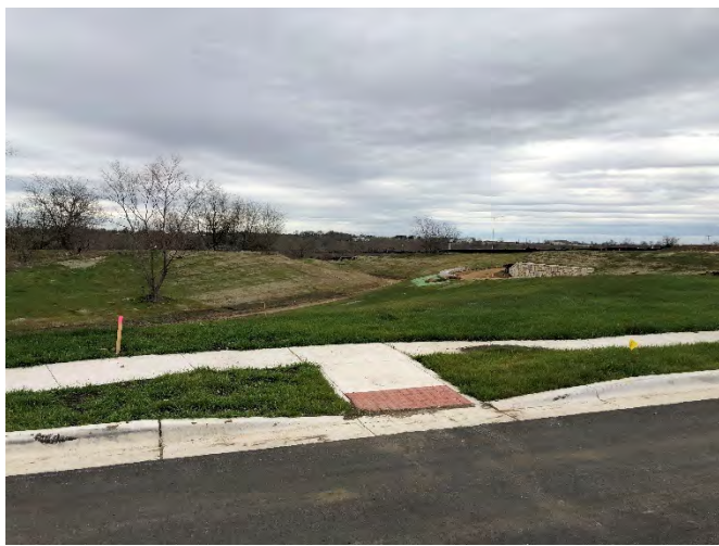
View of completed improvements in Phase I
