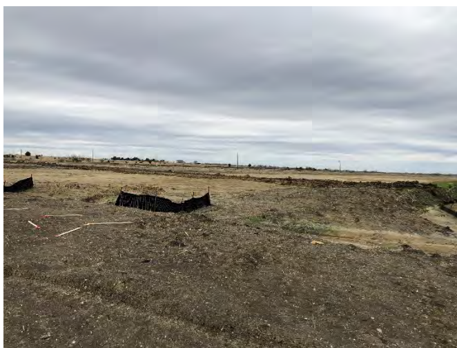
Land under construction in Phase II
