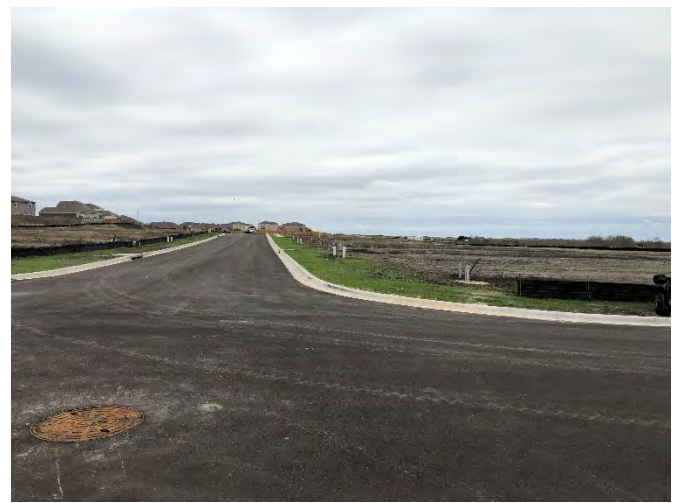
View of completed improvements in Phase I
