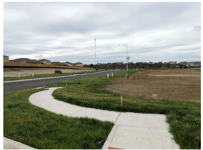
Interior view of improvements in Phase I
