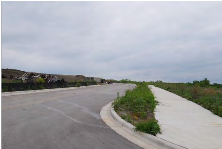
Liberty Bell Boulevard Looking North
