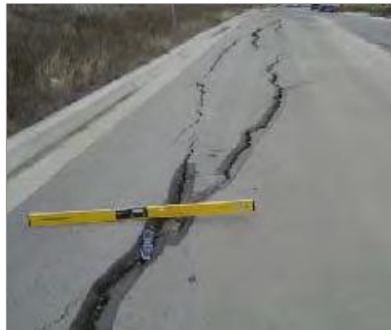
Left: Photo of pavement cracks in a new City of Austin subdivision in 2009. Right: Longitudinal cracking on Golden Falls Drive in Travis County in 2008. Photo credit: City of Austin.
