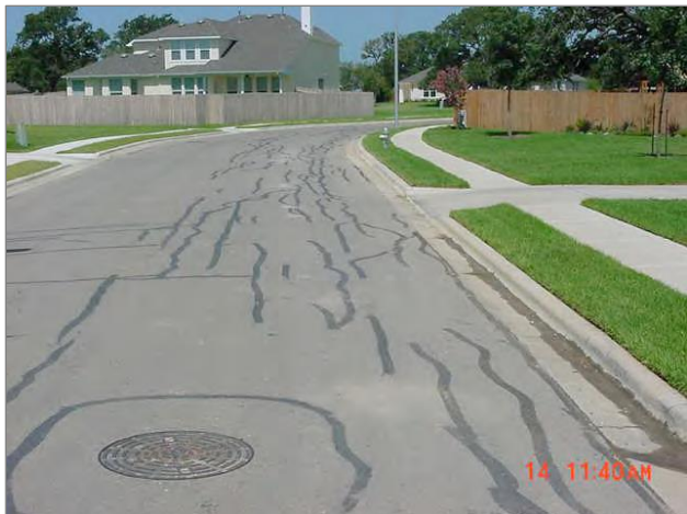
Left: Photo of pavement cracks in a new City of Austin subdivision in 2009. Right: Longitudinal cracking on Golden Falls Drive in Travis County in 2008. Photo credit: City of Austin.
