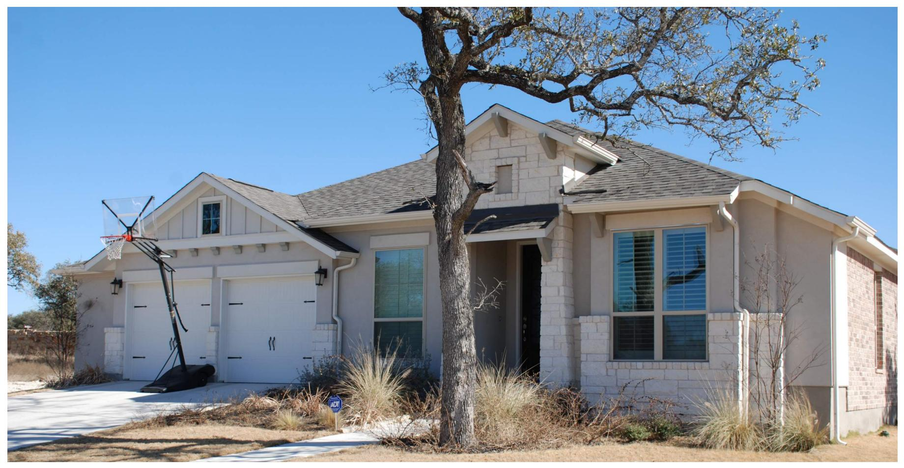
**Materials.** Exterior surface area (all stories) may consist of ledge stone, fieldstone, cast stone, cementious-fiber planking and board and batten (not panels), painted or tinted stucco and brick. Solid wood planking, decorative cementious-fiber panels, galvanized metal and other durable materials may be used for accent features. The minimum front facade masonry is 30%, masonry must be stone, brick or stucco.
