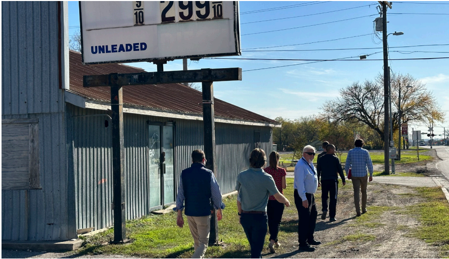
Lack of sidewalks. Lack of building maintenance. Overhead utilities.
