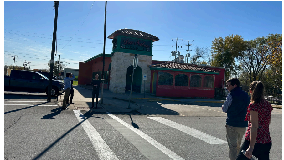
Lack of sidewalks. Lack of building maintenance.
