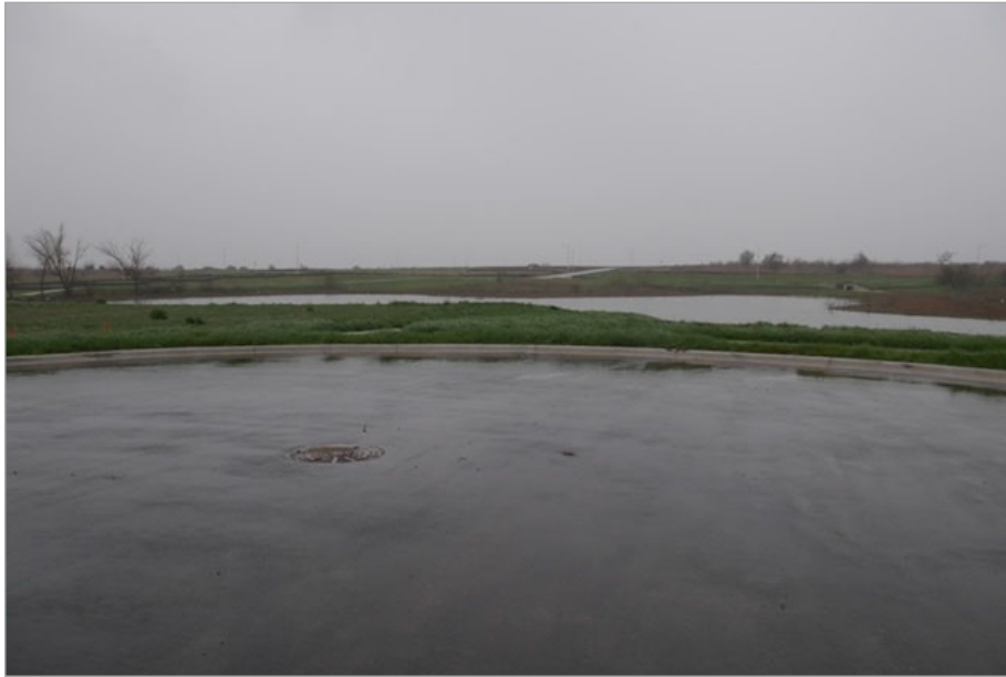
Drainage Pond From Cassidy Lane – Phase 4 Section A
