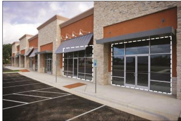
Figure F: The window area is illustrated within the dashed line area for the two storefronts in the above image.
