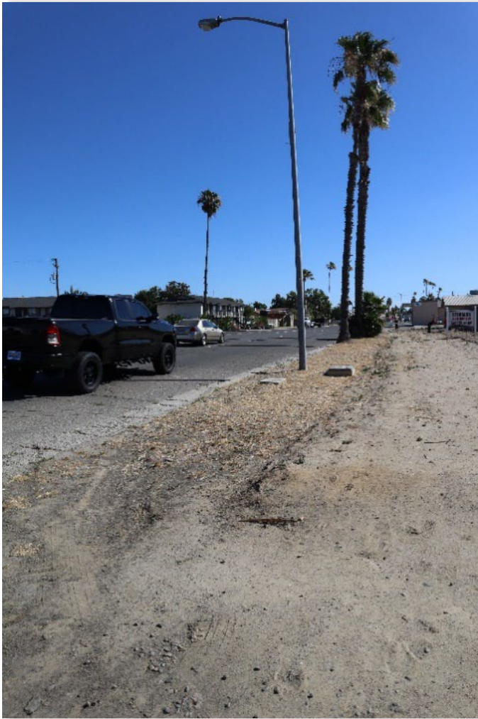
Figure 10: Non-existent sidewalk south of Washington Rd
