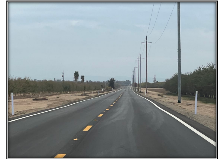
Avenue 26/Road 29 Rehabilitation
