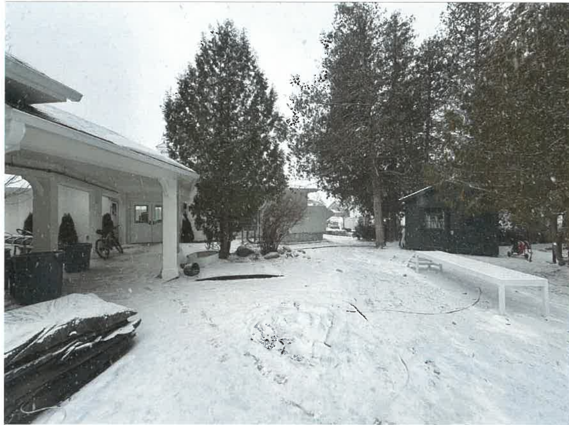
EVENT CENTER SHED
