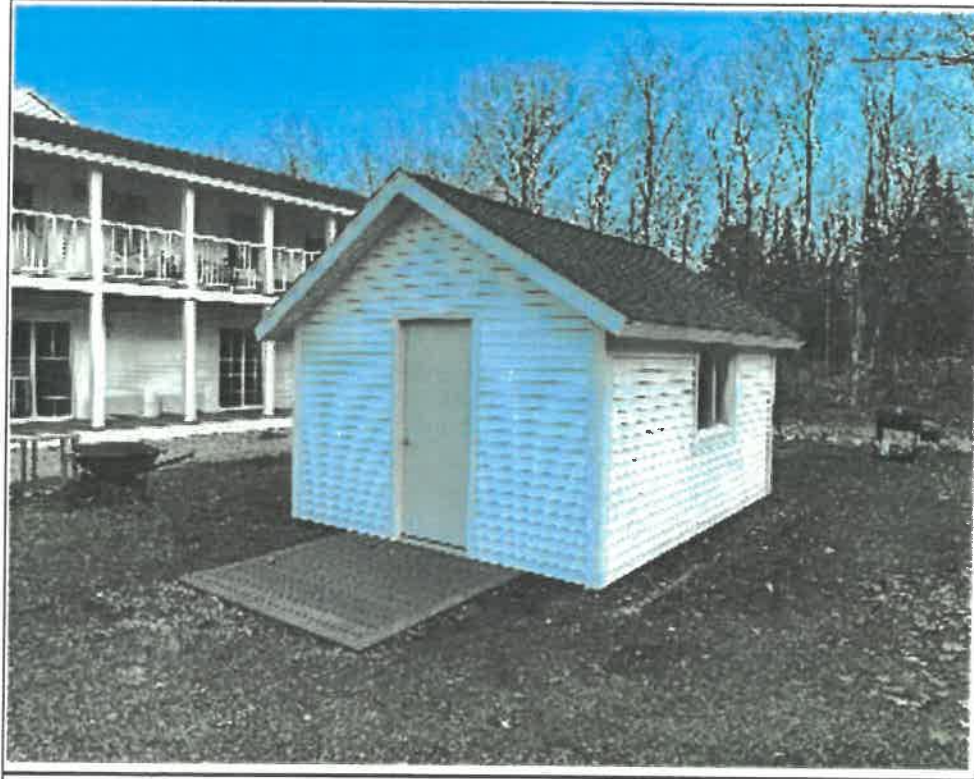
LOOKING EAST AT SHED FROM LOT
