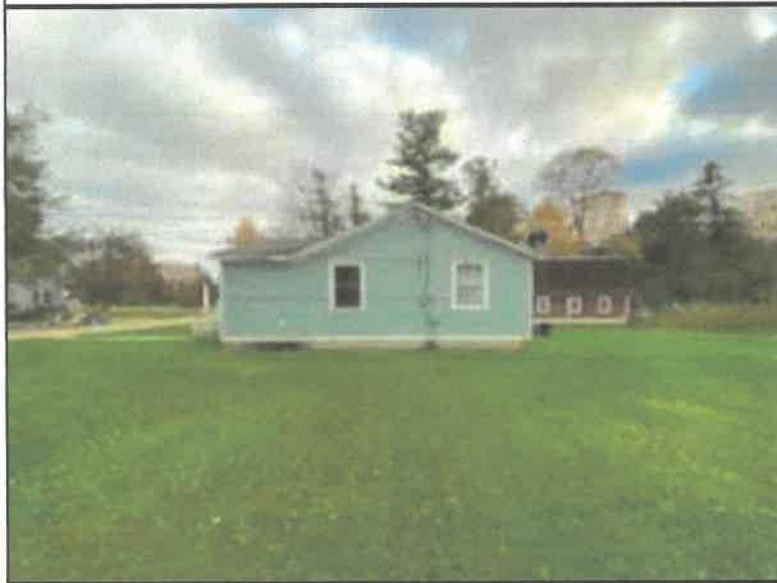
Existing House North
