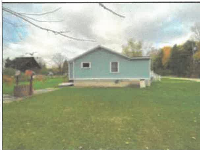
Existing House South
