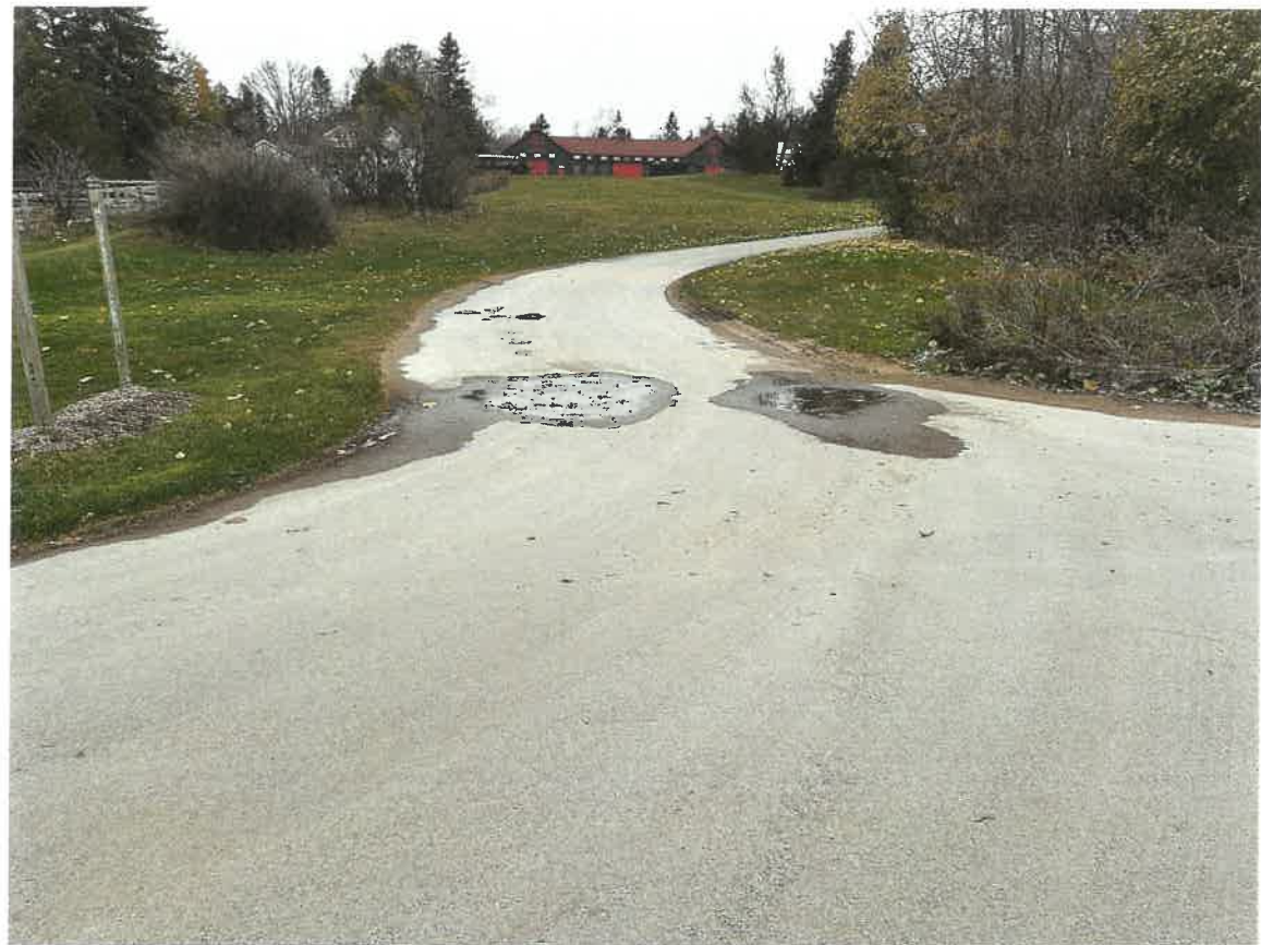
PHOTOGRAPH | LOOKING NORTH ALONG BUTTERFLY LN (GRAND STABLE)
