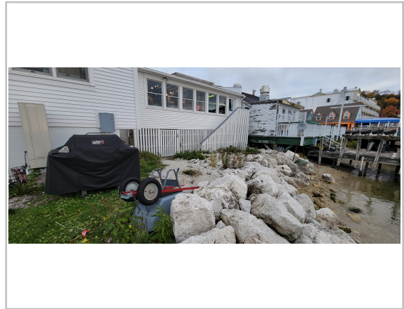
Photo: 14 Looking: N Taken: 10/22/23
