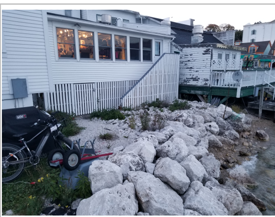
Photo: 17 Looking: N Taken: 10/13/23
