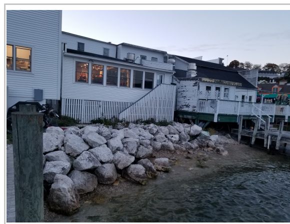
Photo: 18 Looking: N Taken: 10/13/23
