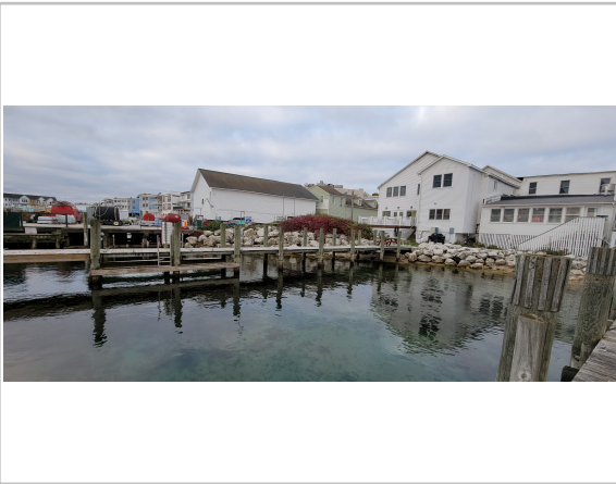
Photo: 13 Looking: W Taken: 10/22/23
