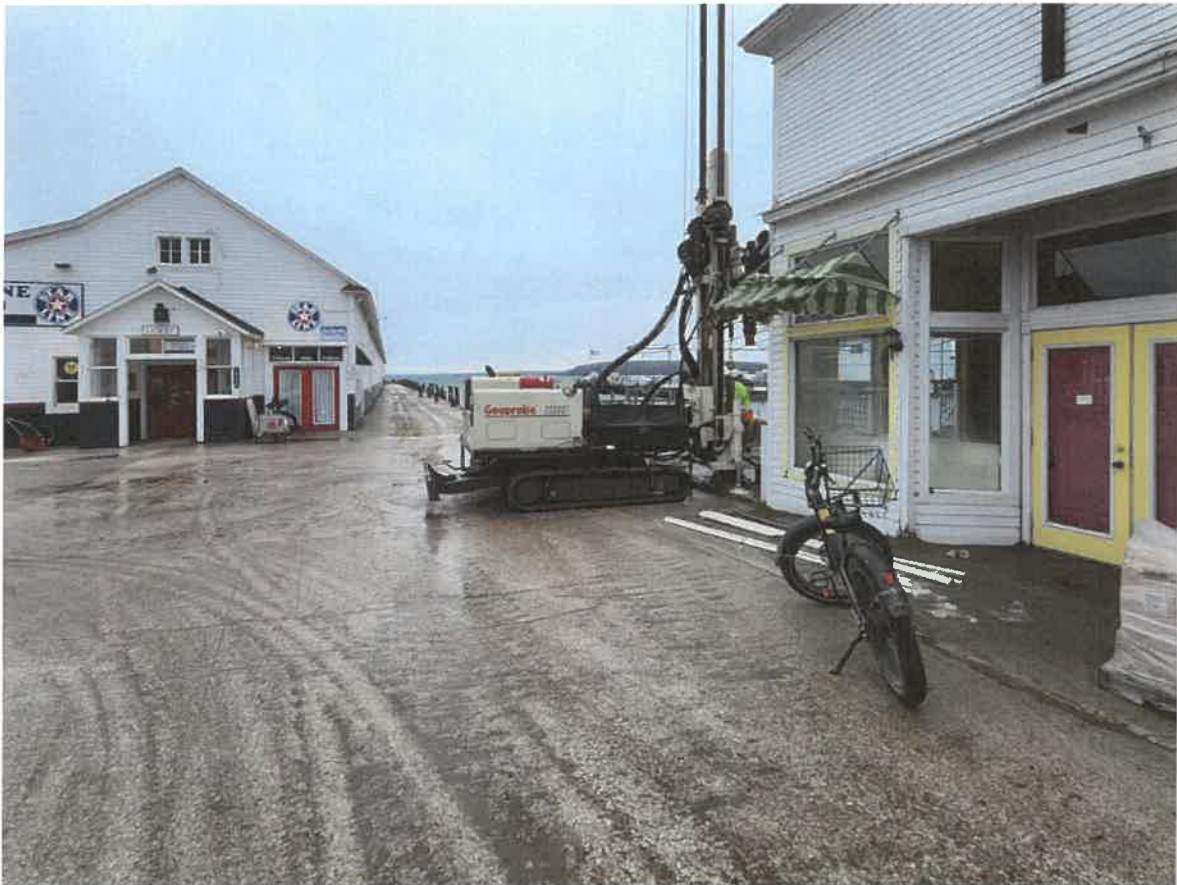
Photograph #1: View of the existing building and concrete dock. The view is to the southeast. [Project No. 2022.2381, Thunderbird Gifts – Deck Settlement, Mackinac Island, January, 2023]
