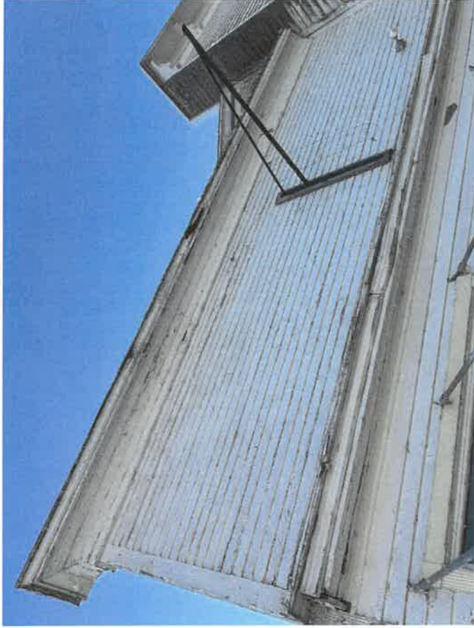
Parapet w/ Top & Intermediate Cornices
