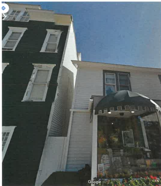
1417 HOBAN STREET, PARTIAL SOUTH FACADE
