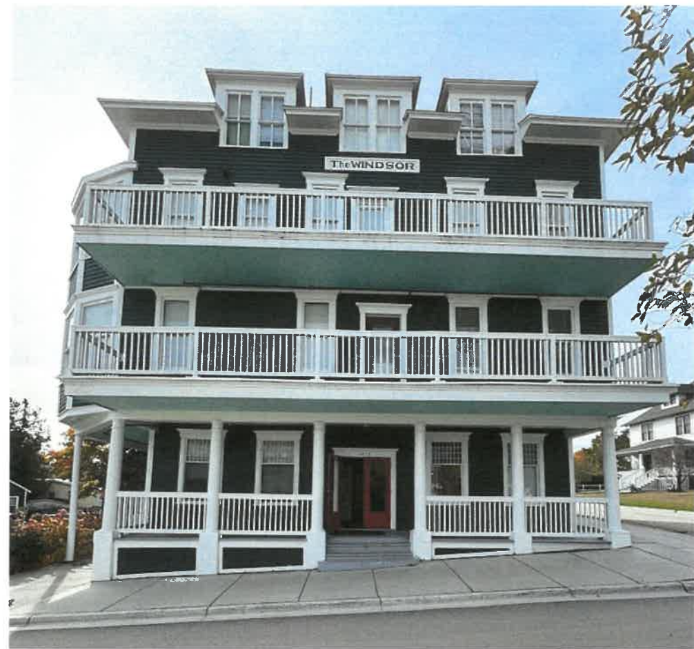
1417 HOBAN STREET, NORTH FACADE
