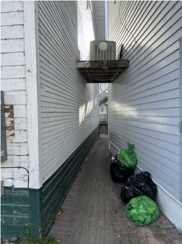
ALLEY FROM DISCHARGE SIDE
