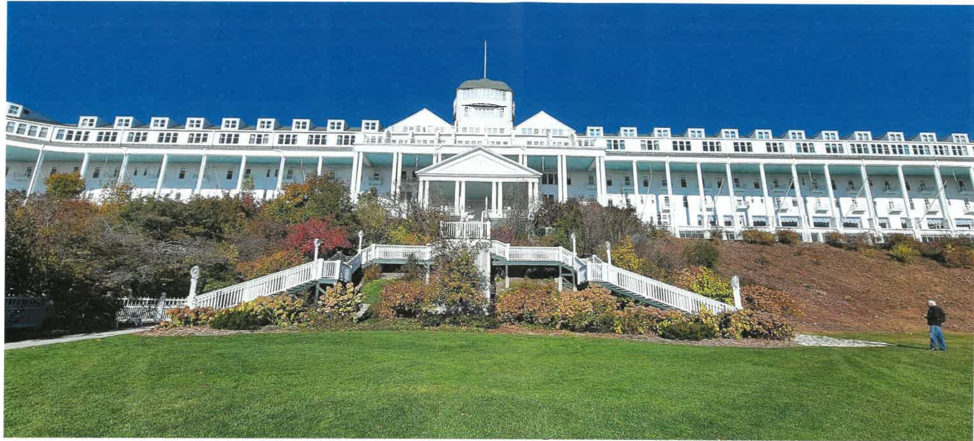
STAIRS LOOKING NORTH
