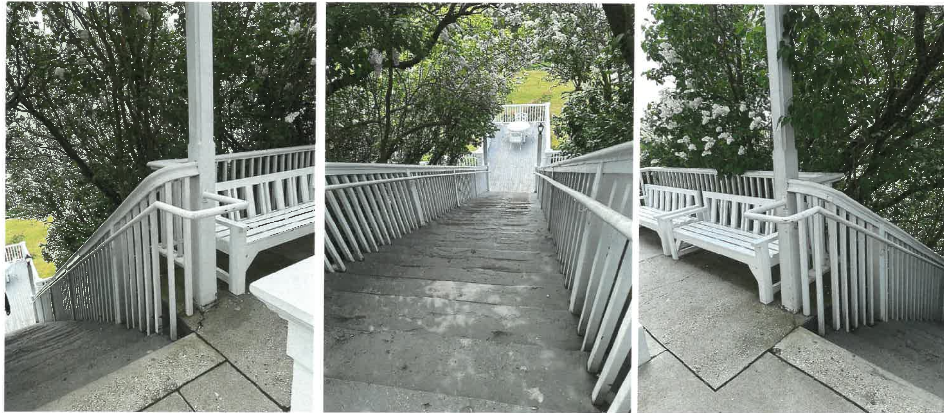
TOP OF STAIRS LOOKING SOUTH
