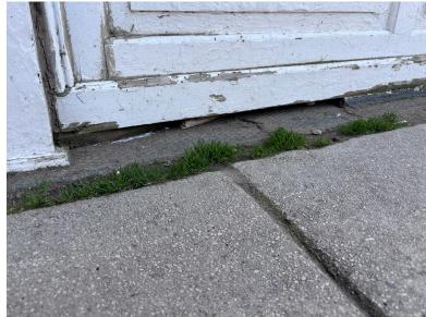
New Wood trim and panels would match current style. Rot and broken pieces would be replaced.
