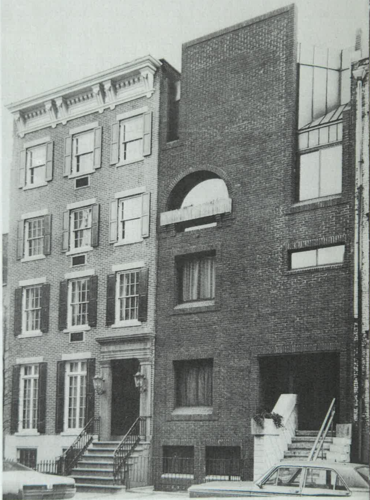
In renovating the mid-19th Century row house in New York's historic Chelsea section, the architect gained an
