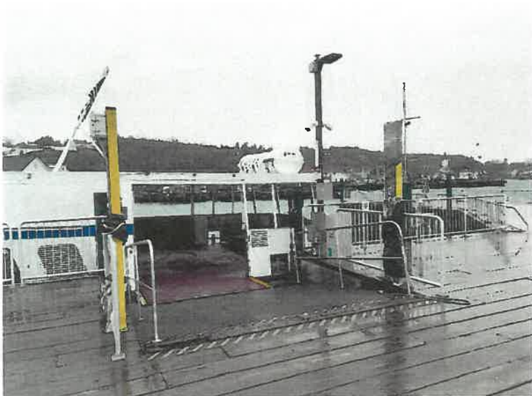
Ramp 3 Picture taken 3.26.24
