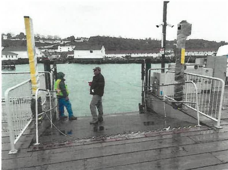
Ramp 2 Picture taken 3.26.24
