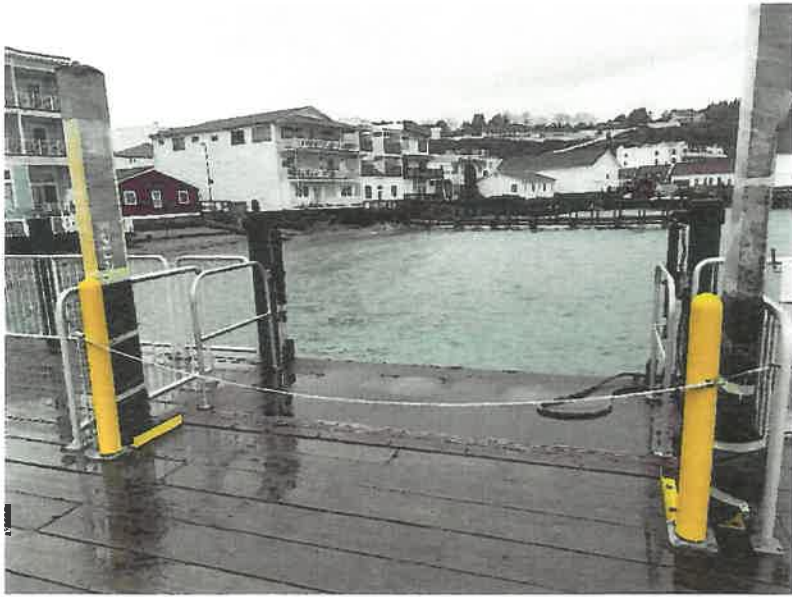
Ramp1 Picture taken 3.26.24
