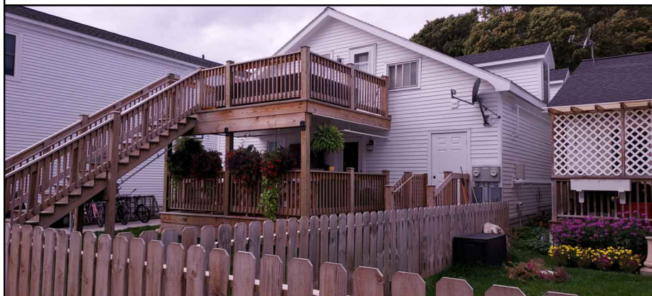
ALLEY VIEW OF GULL
