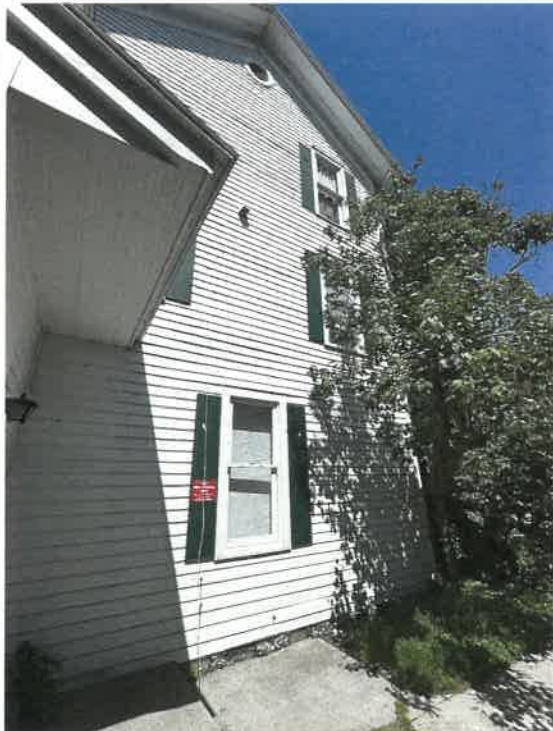
EAST ELEVATION - PHOTO C
