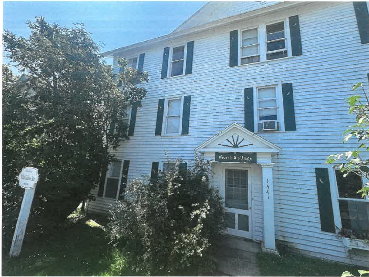
NORTH ELEVATION - PHOTO A
