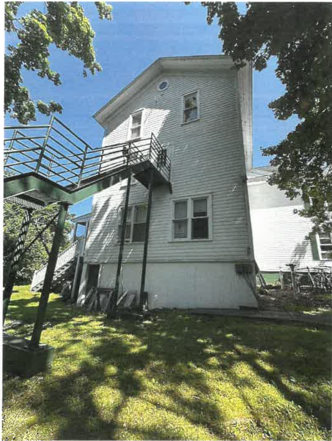
SOUTH ELEVATION - PHOTO H
