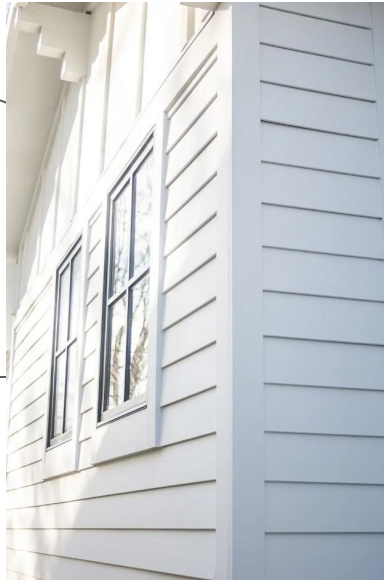
Cladding: LP SmartSide , "Brushed Smooth" finish Trim: 4", 10" Corner boards Rake Water Table Vertical siding: 16" Lap siding: 6" (4" reveal)
