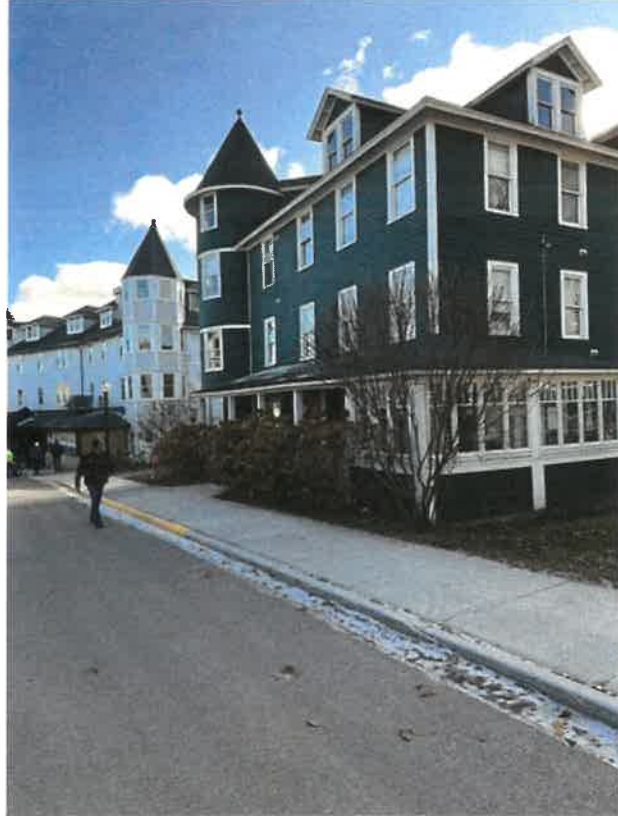
STREET FRONT OF BUILDING, LOOKING SOUTH
