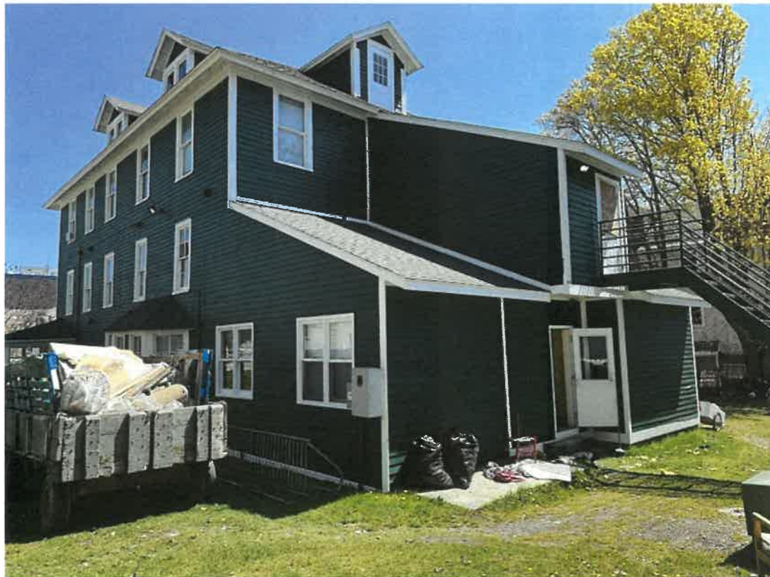
REAR OF BUILDING, LOOKING EAST
