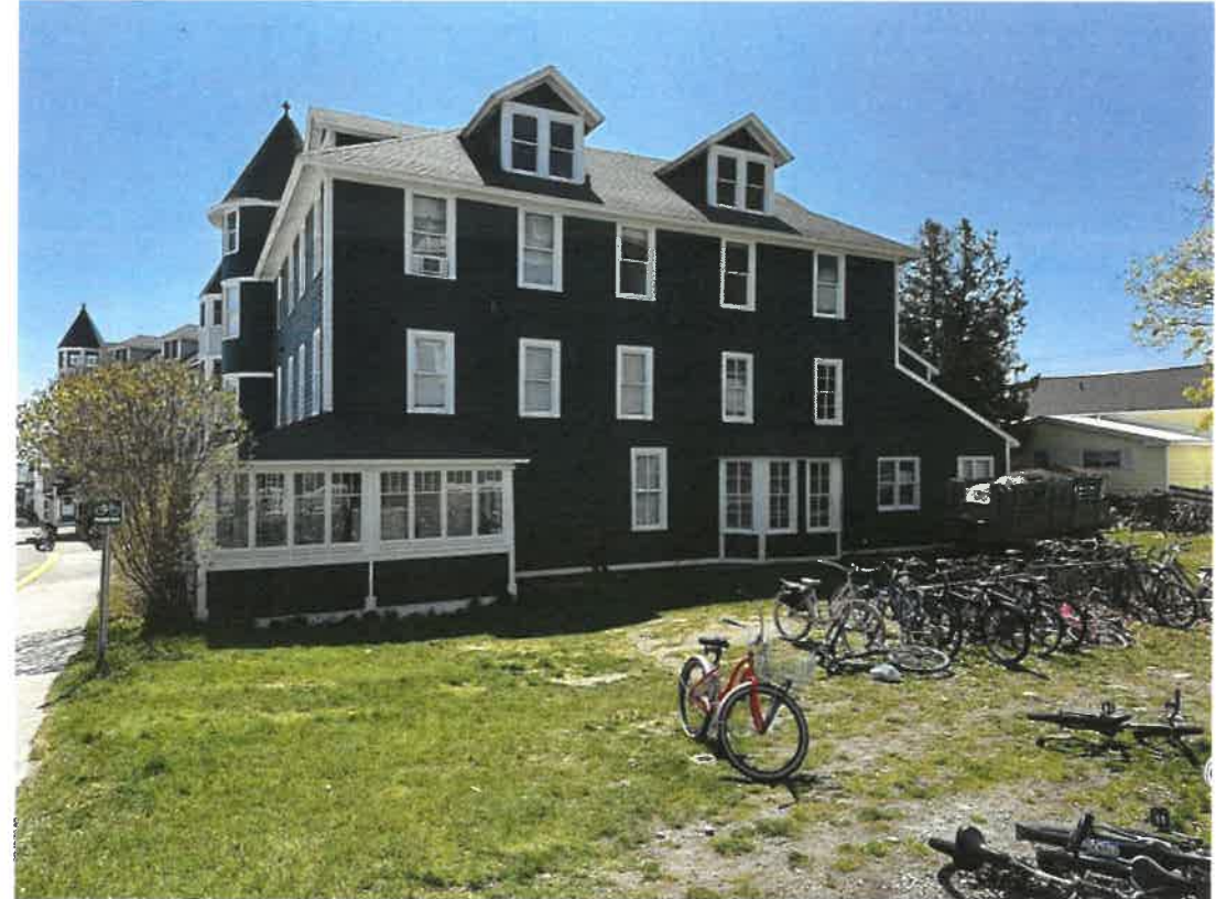
SIDE VIEW OF BUILDING, LOOKING SOUTH-EAST
