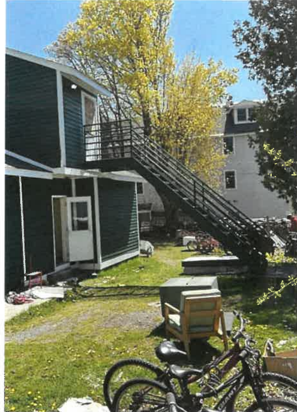
REAR EGRESS STAIR, LOOKING EAST
