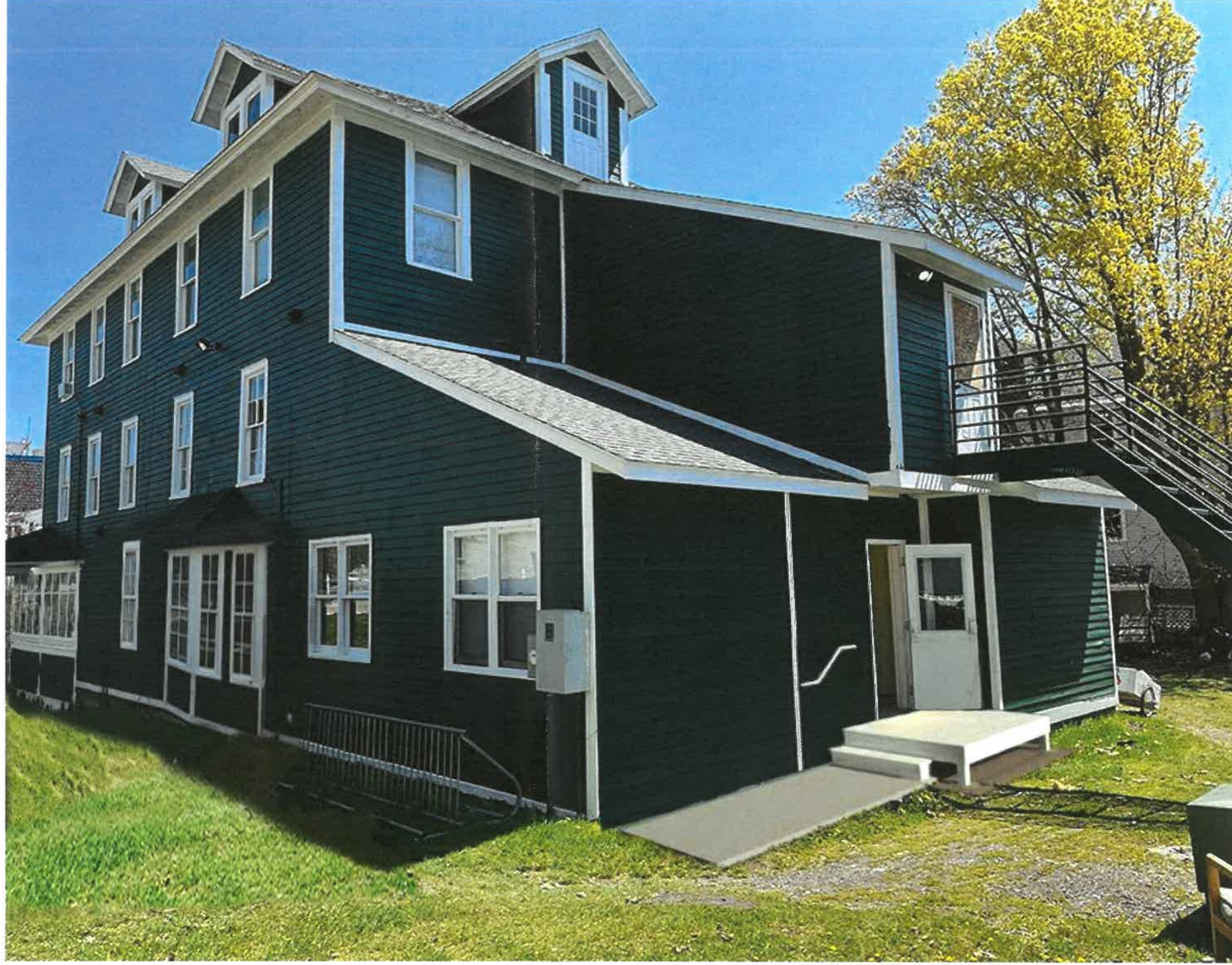
VIEW OF NEW CONSTRUCTION - REAR EGRESS PORCH, LOOKING EAST
