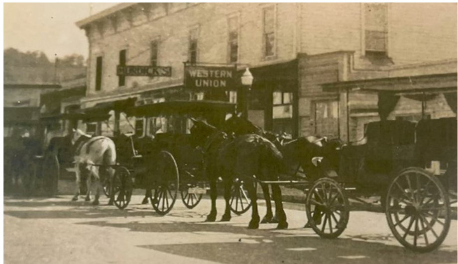
Figure 1-6. Similar view looking northeast at Main Street from closer to Hoban Street, with the subject building on the right. Again the Western Union sign is visible, but the building to the south has changed. Ca. 1920 (Mackinac State Park Archives).
