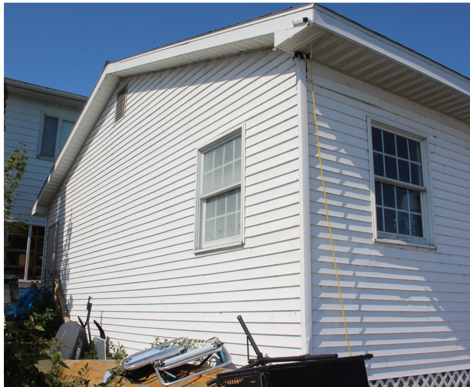
CORNER OF EXISTING SHED, LOOKING NORTHEAST
