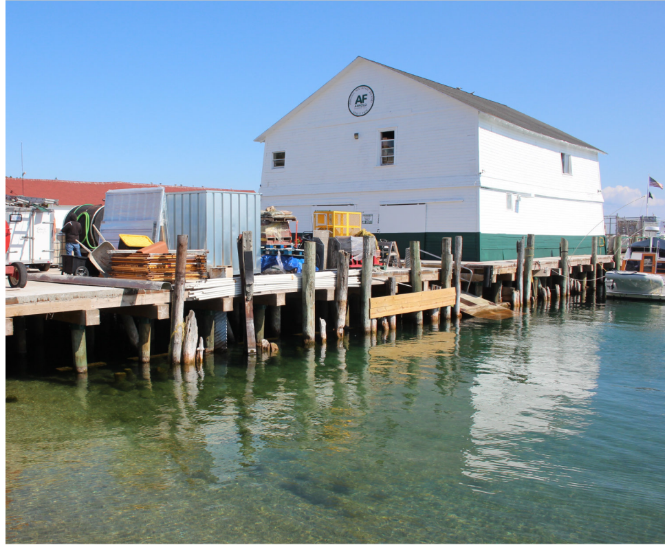
NEIGHBORING BUILDING, LOOKING SOUTHEAST FROM DECK
