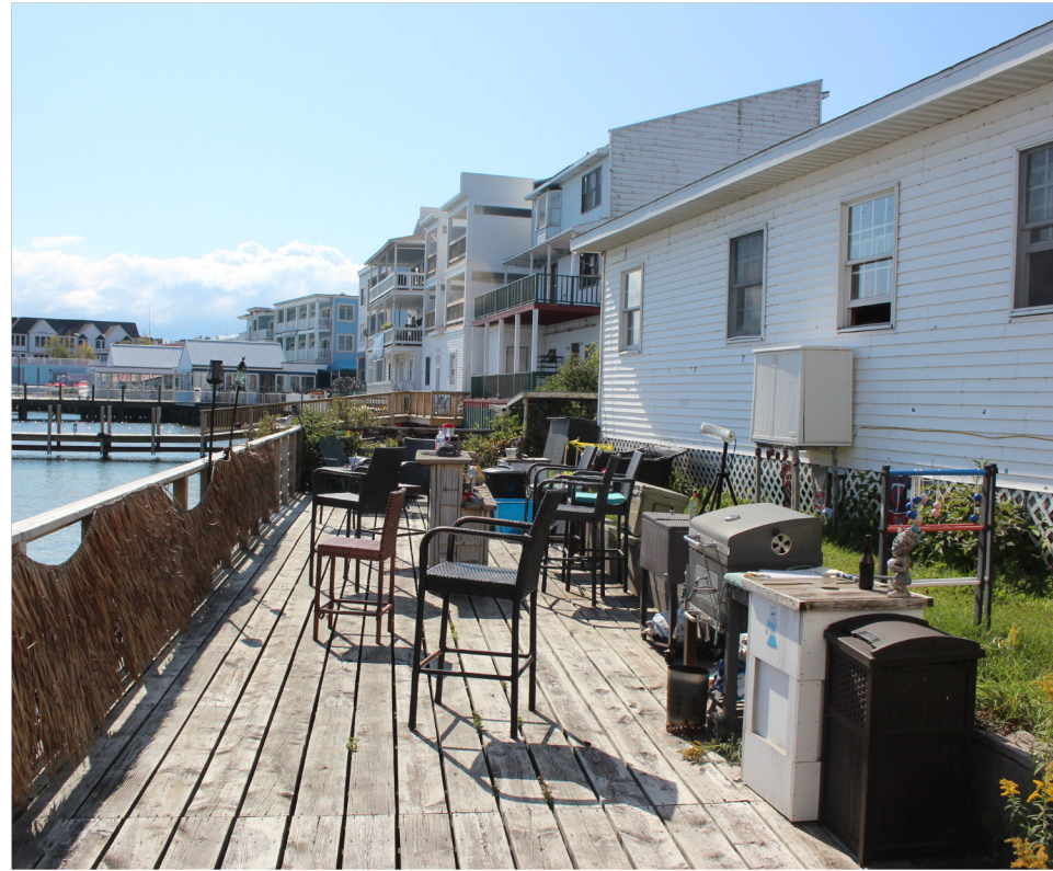
EXISTING DECK SOUTH OF SEA WALL, LOOKING WEST
