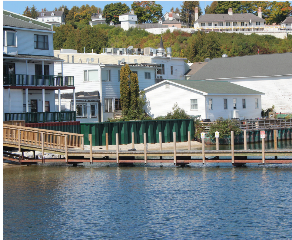
EXISTING BUILDING, SHED AND SEAWALL, LOOKING NORTHEAST
