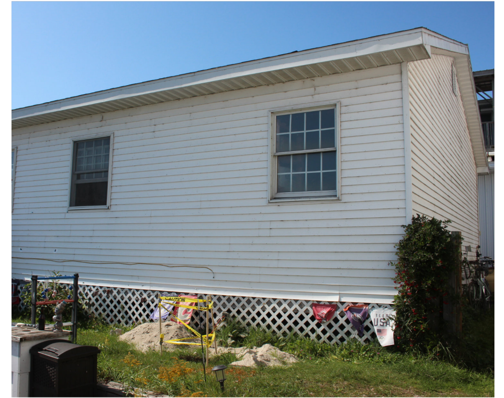
CORNER OF EXISTING SHED, LOOKING NORTHWEST
