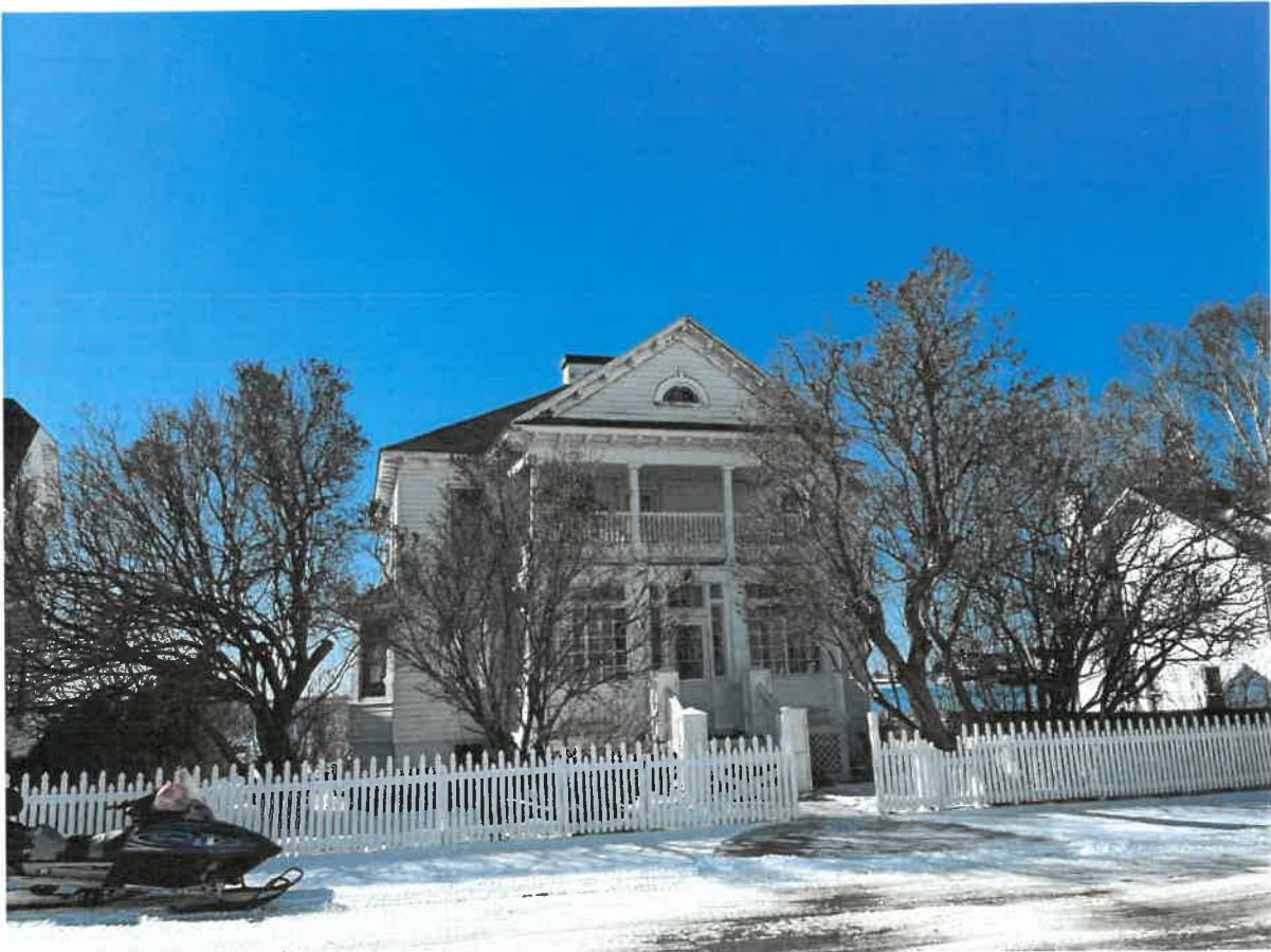
Photo 5. Saint Anne's Rectory, 6837 Main Street
