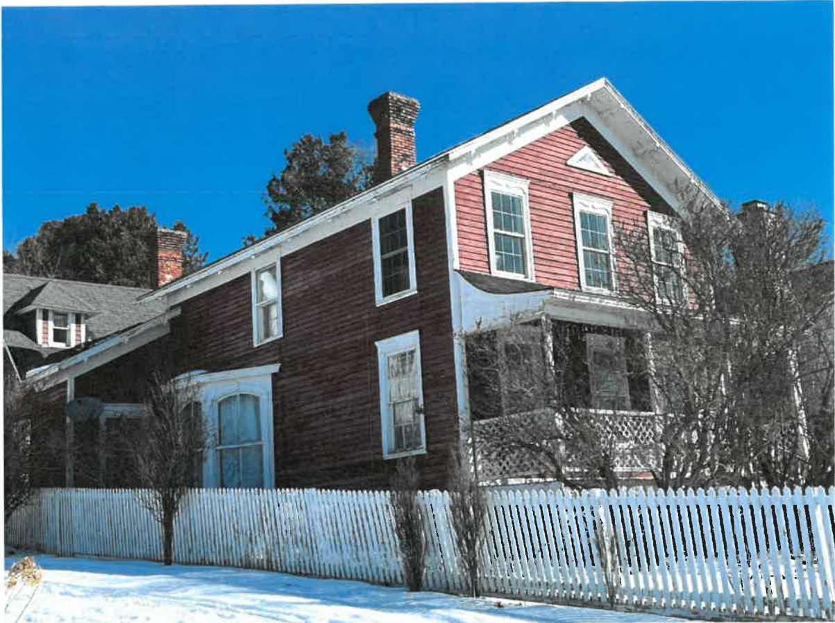
Photo 2. 6948 Main Street, c. 1850.
